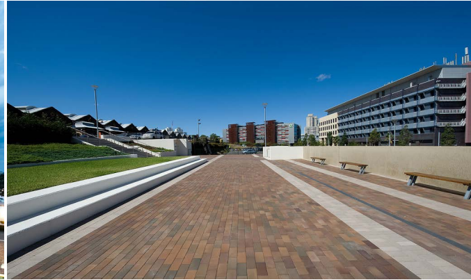
3. Biomedical building (1 Central Avenue) - to right
