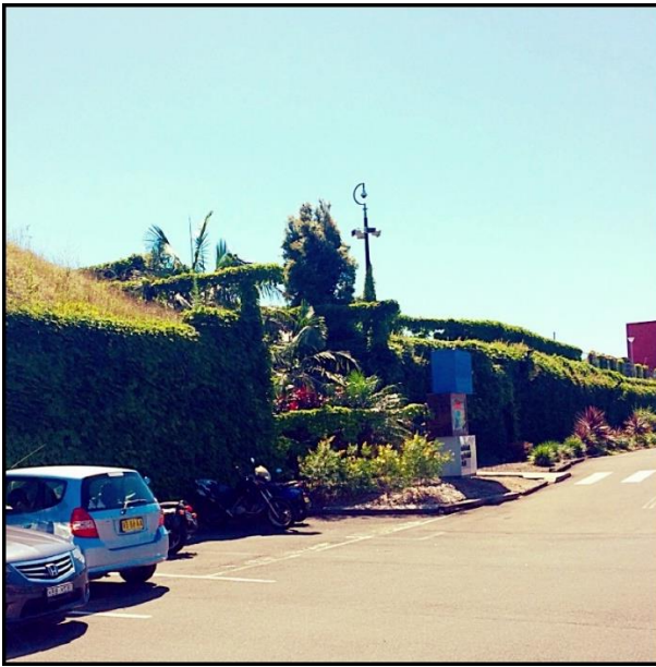
FIGURE 4: IVY COVERED FOUNDRY WALLS
