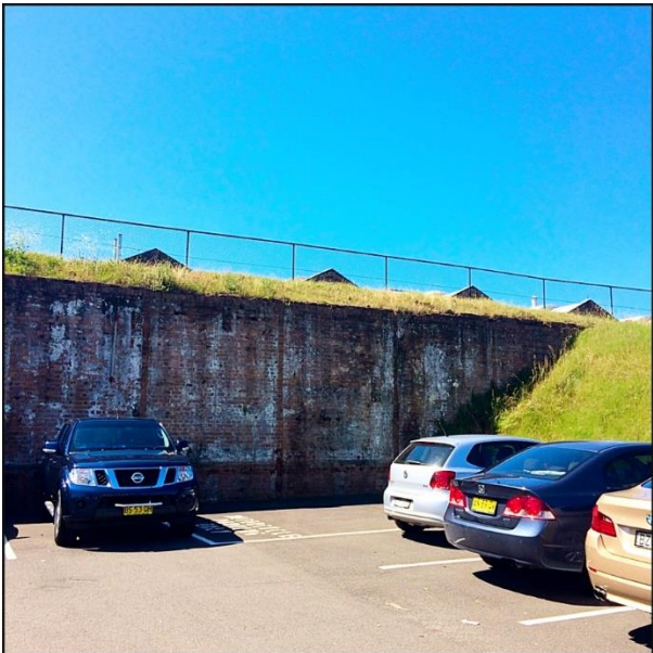
FIGURE 6: VIEW OF FOUNDRY WALL LOOKING NORTH.
