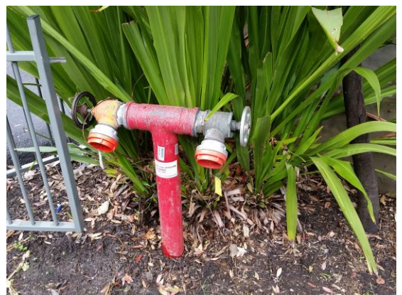
Typical twin head pillar hydrant
