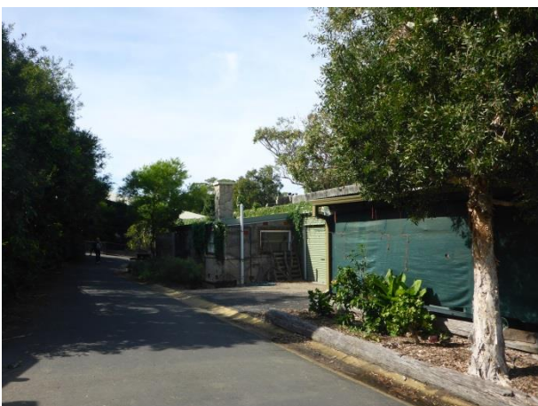
PICTURE 5 – VIEW OF THE REAR (NORTHERN) FAÇADE OF THE FSAB AND ADJOINING 'FEMALE AMENITIES BUILDING', FACING WEST
