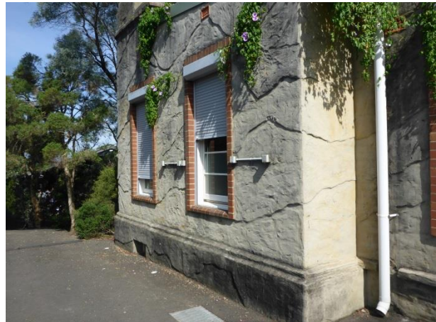
PICTURE 4 – VIEW OF THE EASTERN FAÇADE OF THE BUILDING, FACING SOUTHWEST
