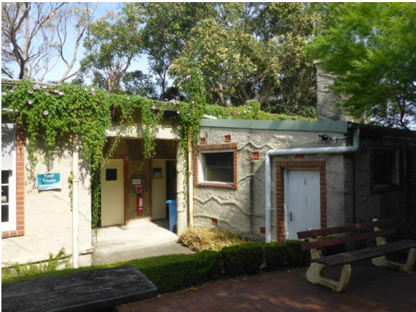
PICTURE 3 – VIEW OF THE REAR (NORTHERN) FAÇADE OF THE BUILDING, FACING SOUTHWEST
