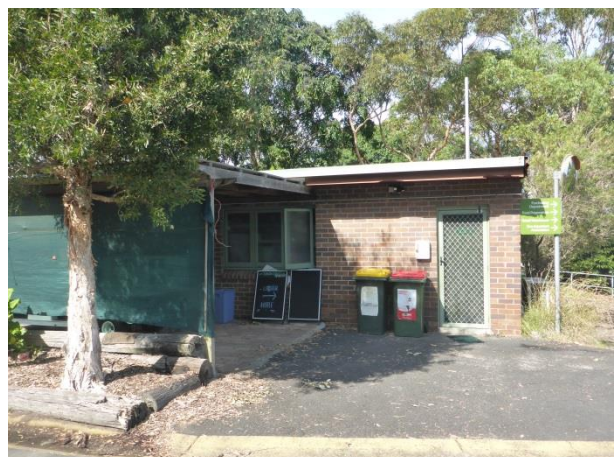
PICTURE 6 – VIEW OF THE REAR FAÇADE OF THE 'FEMALE AMENITIES BUILDING'
