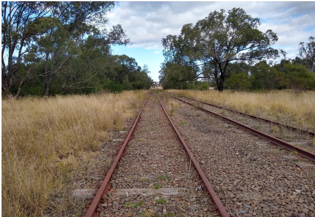
Photo 4 - Central northern portion of railway corridor
