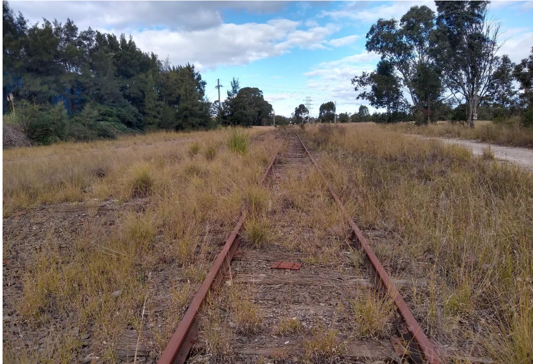
Photo 1 - Northern portion of the railway corridor
