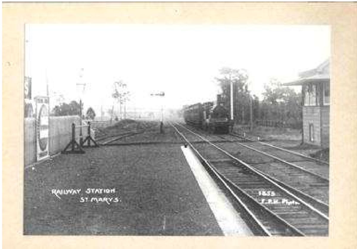
Plate 4. St Marys Railway Station, c.1900s (Image: Penrith City Library).
