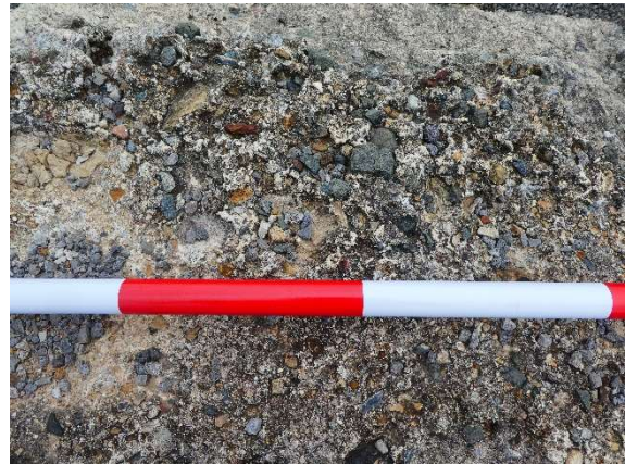
Plate 30. Conglomerate concrete block.
