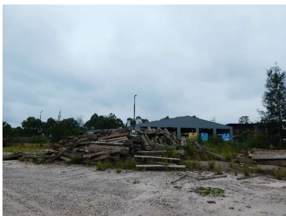
Plate 39. Concrete railway sleepers in piles along the eastern boundary of the site. Bus depot present adjacent to the site.
