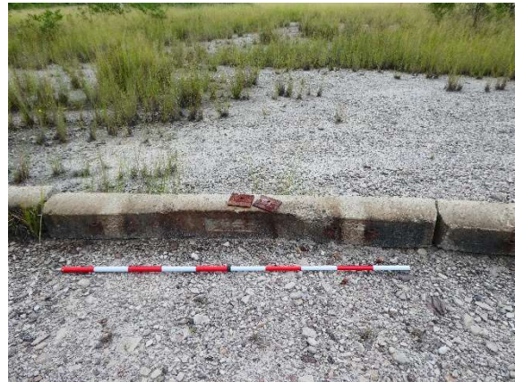
Plate 36. Concrete railway sleeper with two associated metal anchors.
