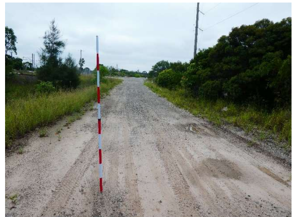
Plate 14. Forrester Road entrance corridor. Facing west towards the Intermodal site.
