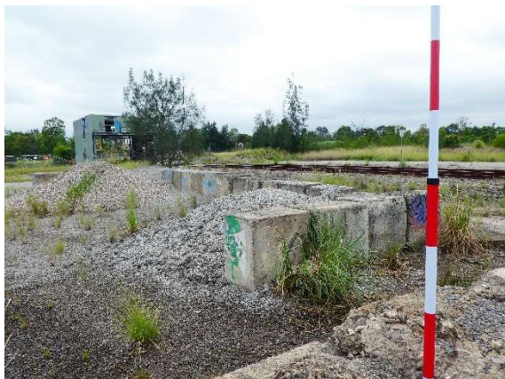
Plate 27. Large conglomerate concrete blocks formed into two 'U' shapes. A significant amount of gravel had accumulated within the form of the 'U'.
