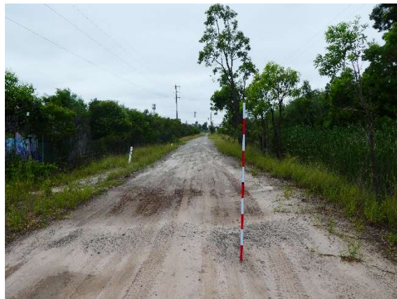
Plate 13. Forrester Road entrance corridor. Facing east towards St Marys Railway Station.
