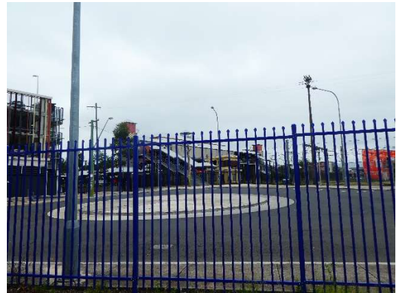
Plate 12. View of St Marys Railway Station from the Forrester Road site entrance. A blue steel fence and locked gate prevent public access to the site.
