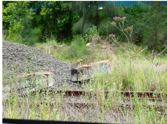
Plate 54. End of railway line in the northern section of the site. A pile of gravel is present immediately north of the end of the tracks. Originally the tracks would have continued further north to the munitions factory railway station.
