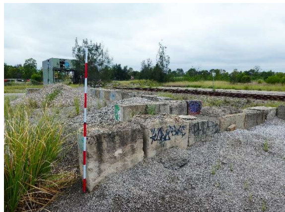
Plate 28. Concrete blocks with graffiti.
