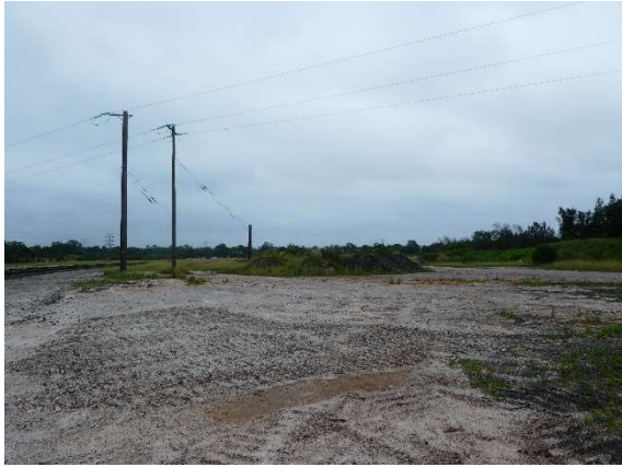
Plate 41. Powerlines running across the site.
