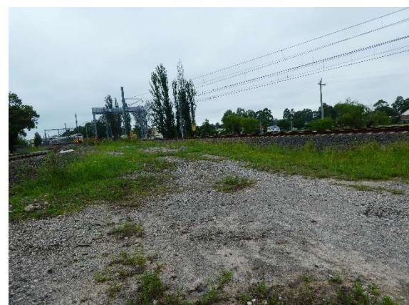
Plate 46. Main Western railway line and St Marys railway station from the southern boundary of the site.
