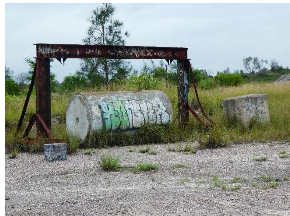
Plate 38. Concrete drum and rusted steelwork with substantial modern graffiti.
