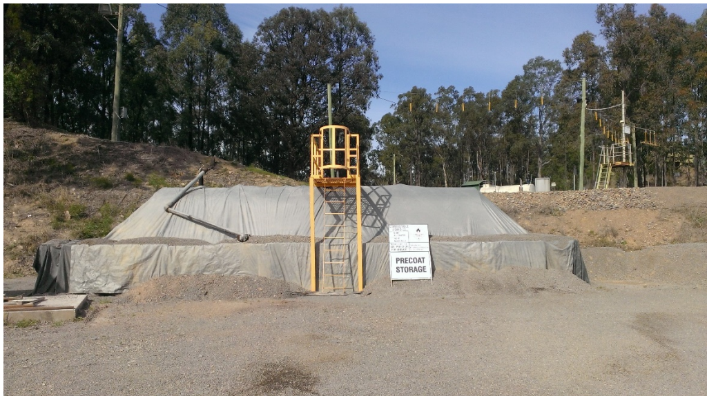
Photograph 15-4 Typical Precoat Supa storage at Sancrox Quarry.
