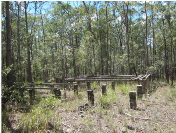
Photograph 11 - Evidence of previous land use - brick piers and timber floor bracing (ERM 2017)
