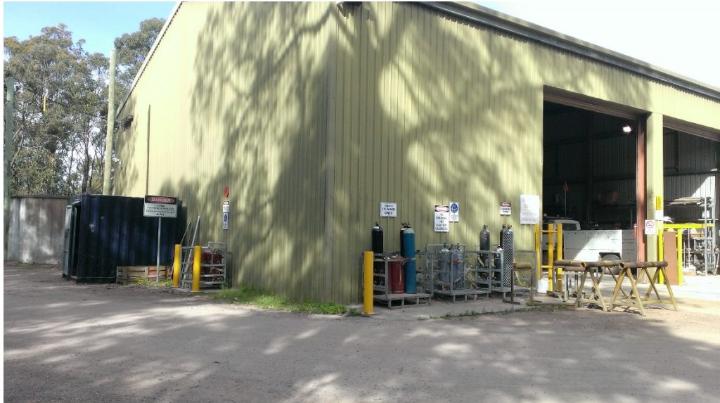
Photograph 15-1 Typical Acetylene and Oxygen storage.
