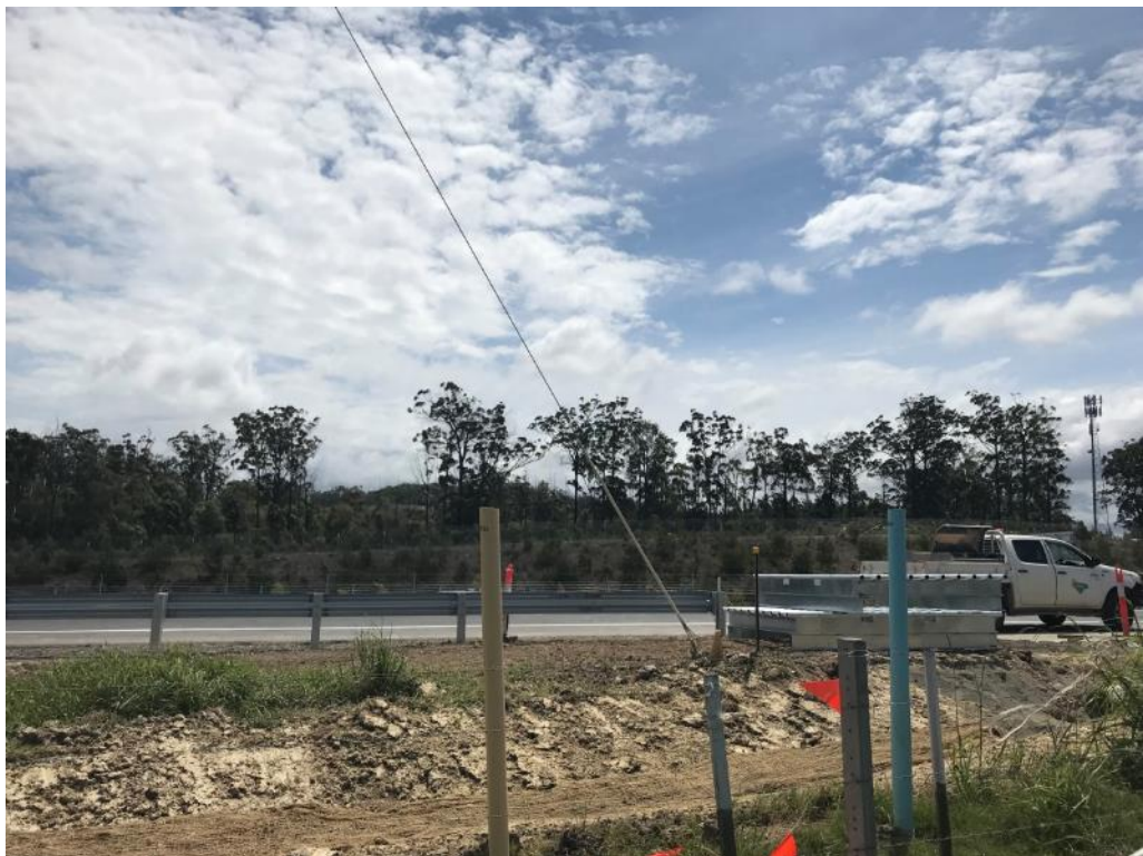
Photograph 6 View from Cassegrain Winery looking west towards the Project site across the Pacific Highway.
