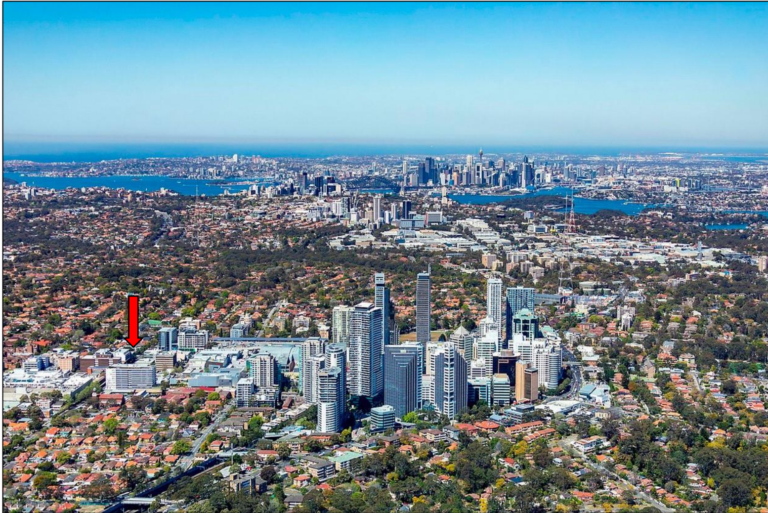
Figure 13: Looking south across the Chatswood CBD skyline and the subject site (red arrow).
