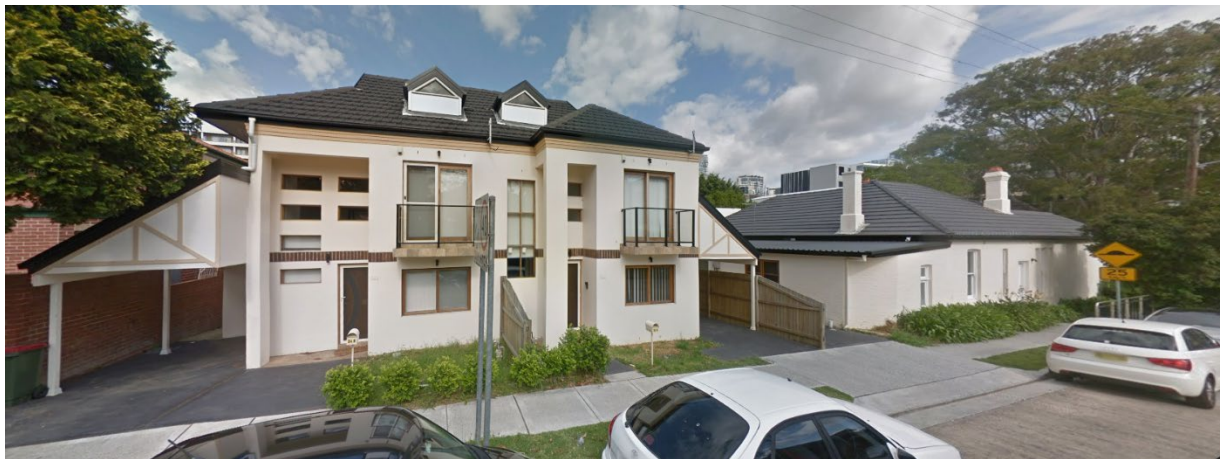
FIGURE 6 – SITE VIEWED FROM BERTRAM STREET LOOKING WEST Source: Google Street View
