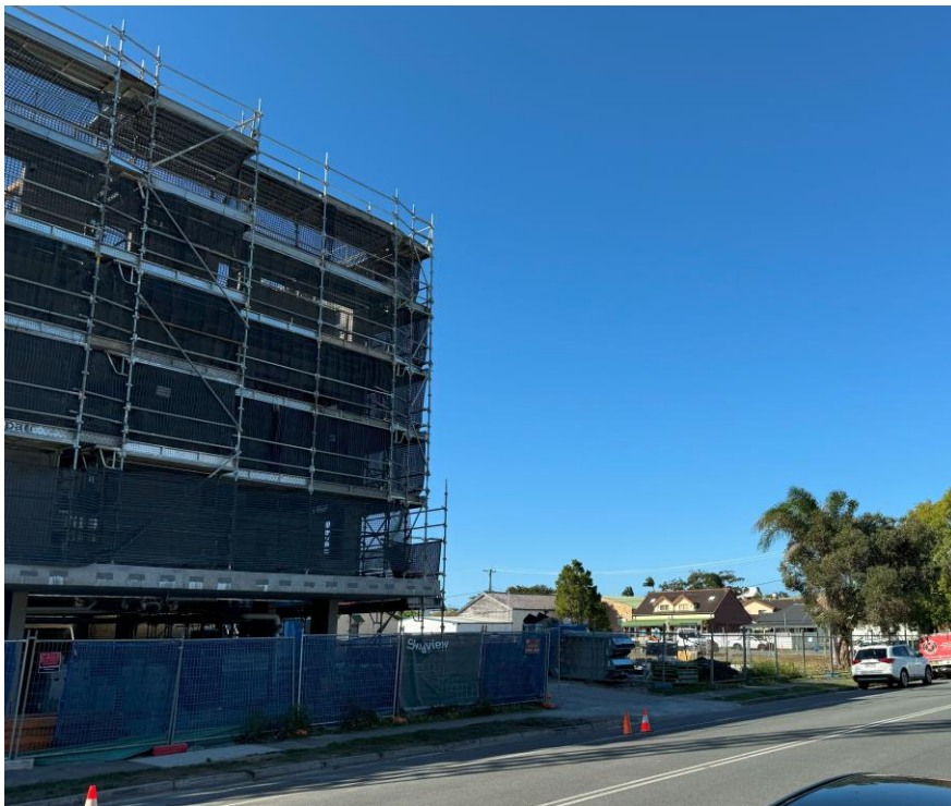
Figure 3 Development at 1 Brett Street under construction adjacent to the site
