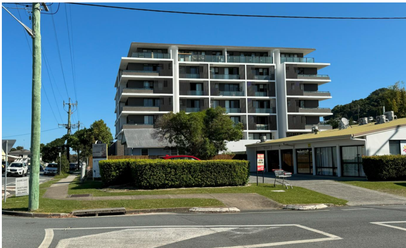
Figure 4 View of the recently completed 33-35 Boyd Street from the Site
