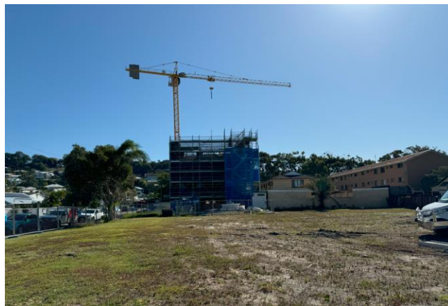
Figure 13 1 Brett/24 Recreation Street under constructed
