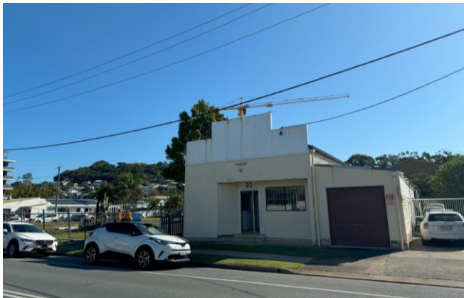
Figure 10 Building at 23 Boyd Street
