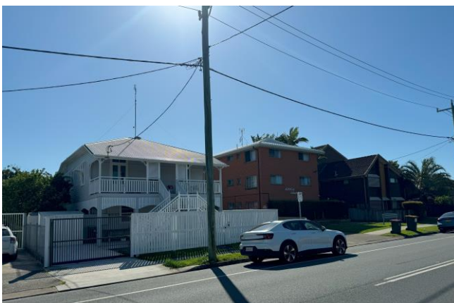
Figure 15 Multi-dwelling housing to the Site's north
