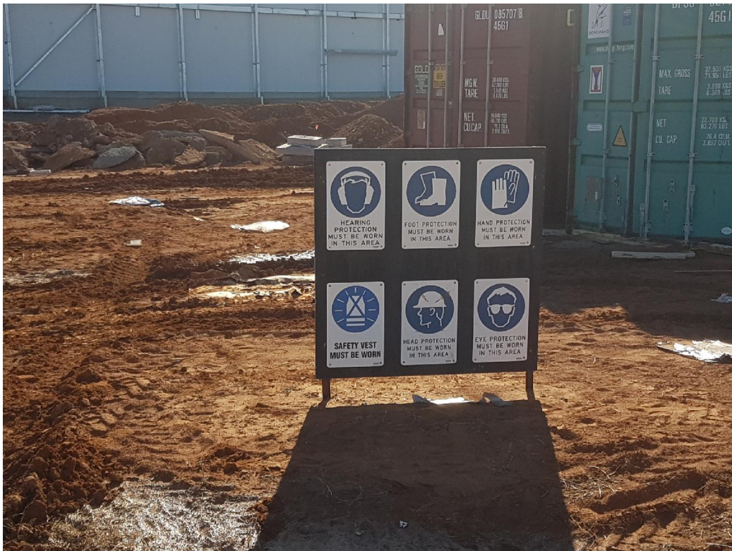
(Photo 6: main construction access signage.)
