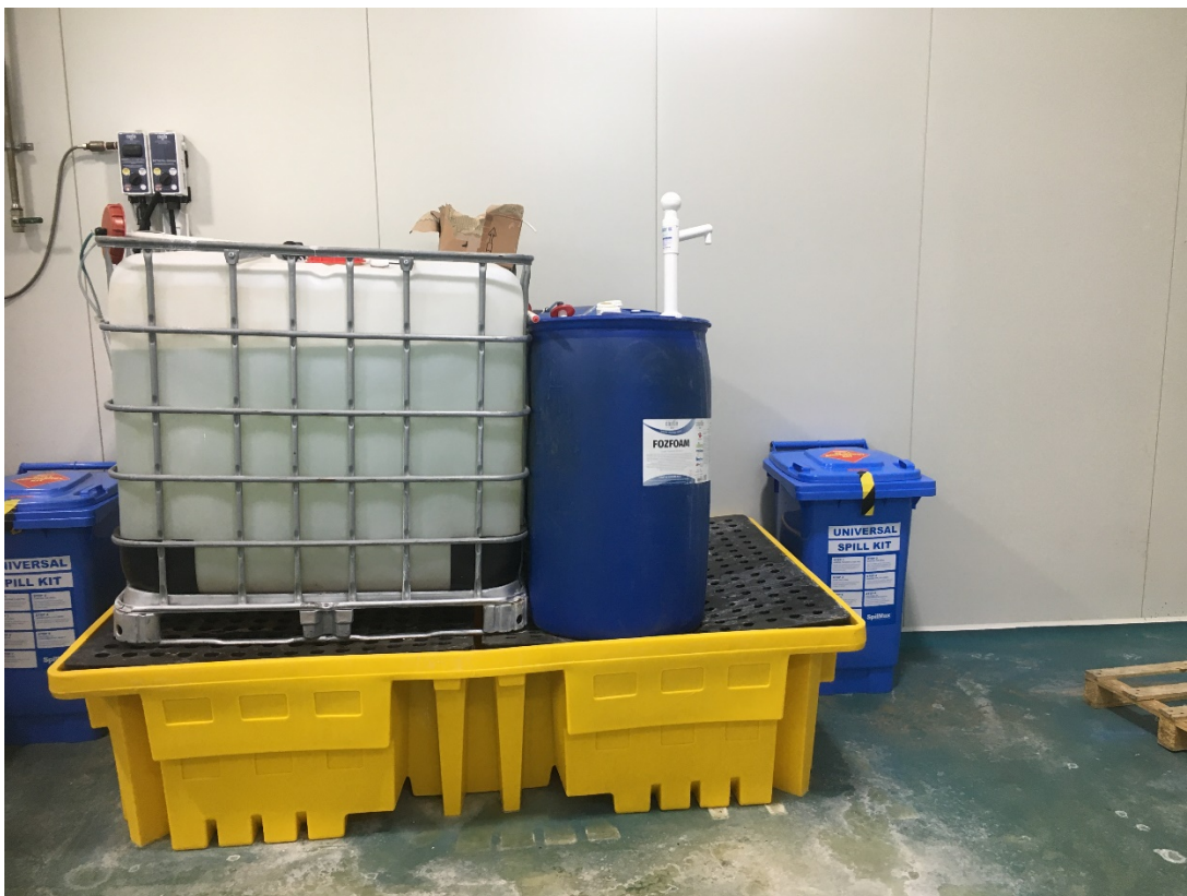
(Photos 1 & 2: banded chemicals and additional spill kits safely stored in chemical room.)
