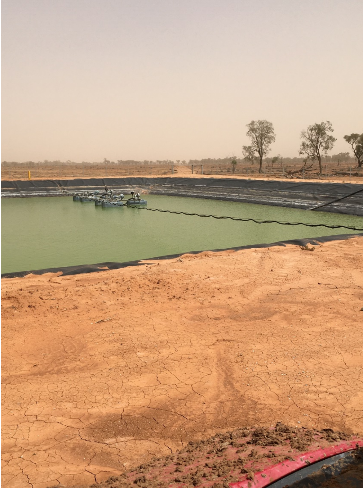
(Photo 16: Wastewater Treatment Pond, Aerator Cables, Anchor Points and fencing from side view.)
