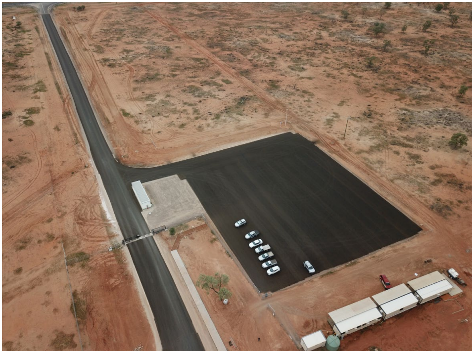
(Photo 14: car park and entrance from main Highway with security gate.)
