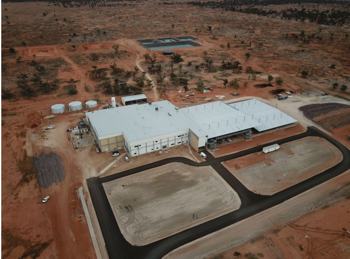
(Photo 13: overview of the Abattoir with mass disposal pit, sealed road and bunded water treatment pond in the irrigation area.)
