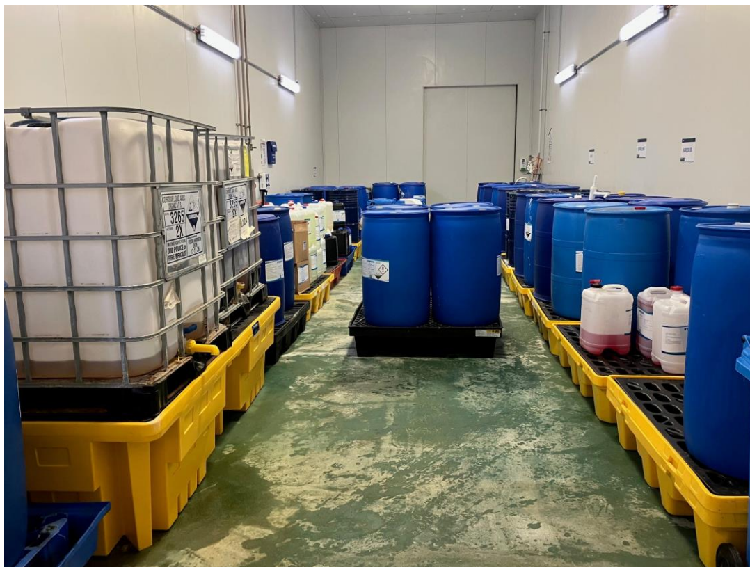
Figure 11: Chemicals kept banded in chemical stores
