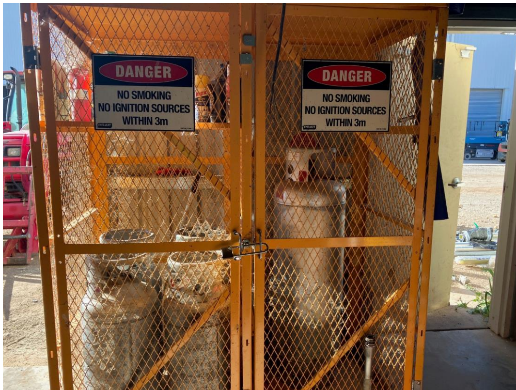
Figure 10: Combustible Chemicals kept bunded and caged
