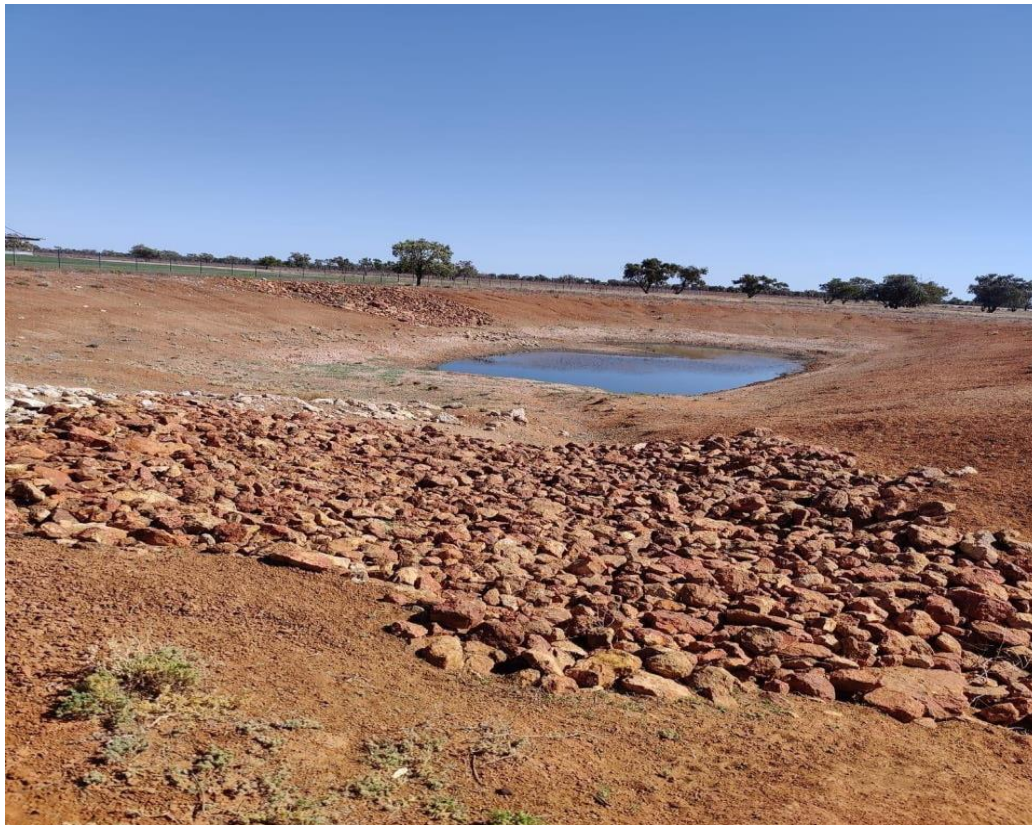
Figure 6: Sediment Dam
