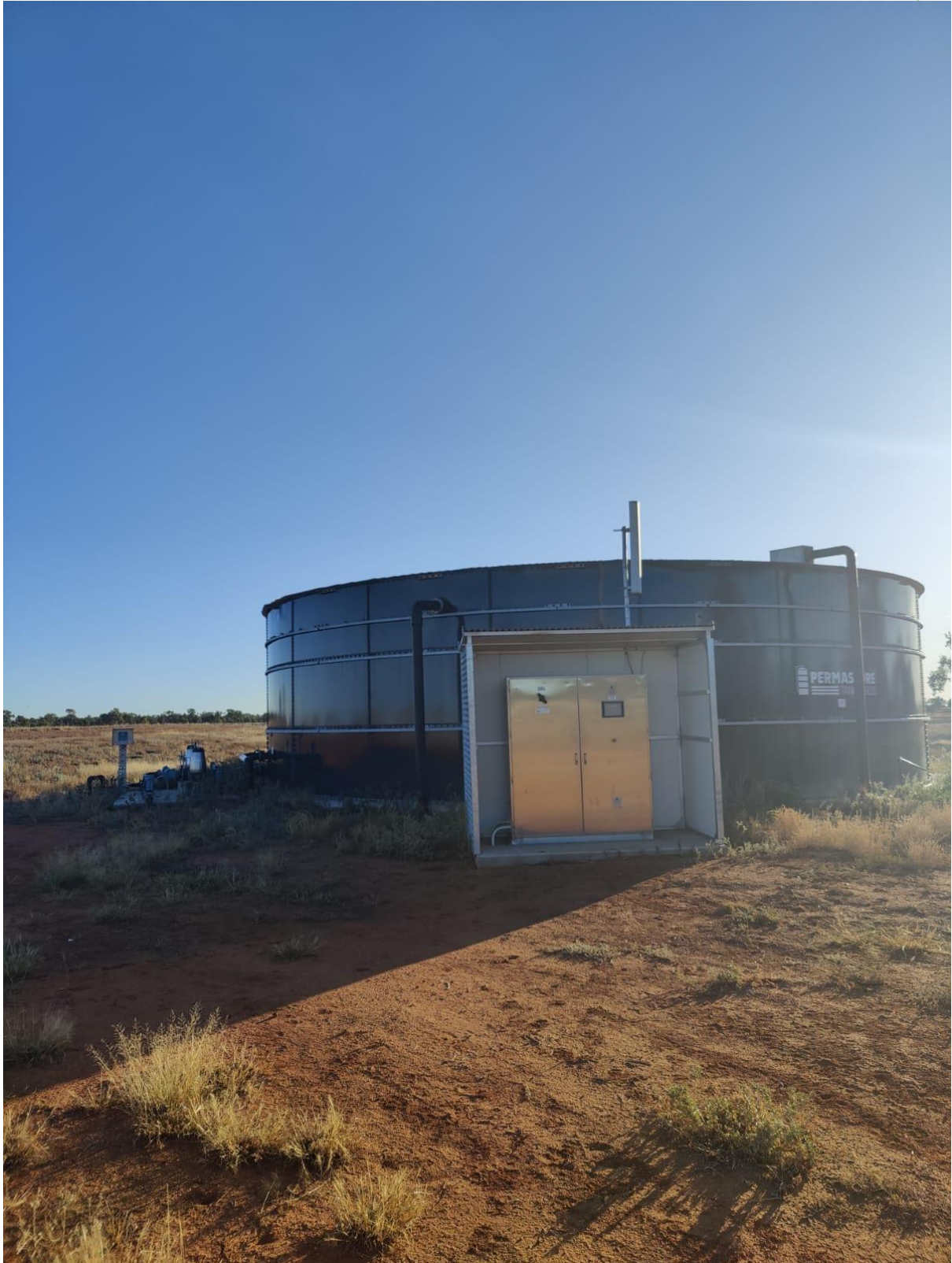
Figure 16: Balance Tank in WWTP Area
