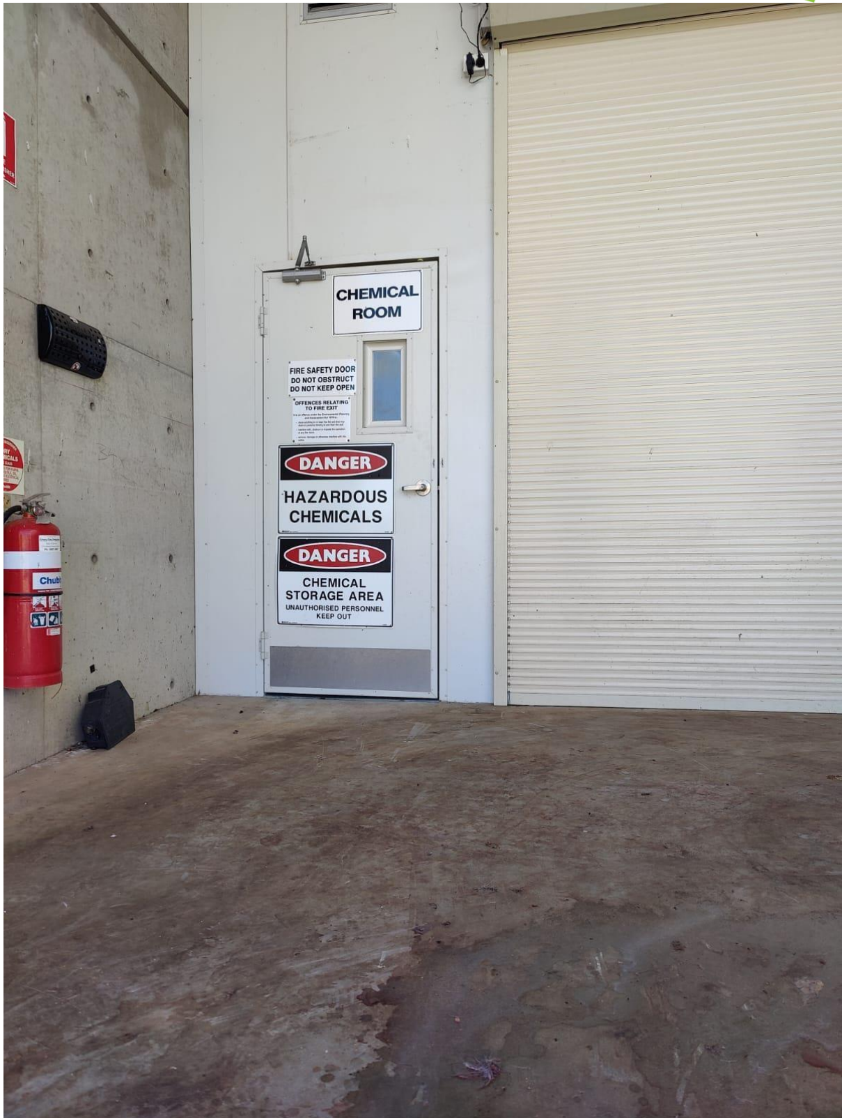
Figure 13: Chemical Room Signage (a)
