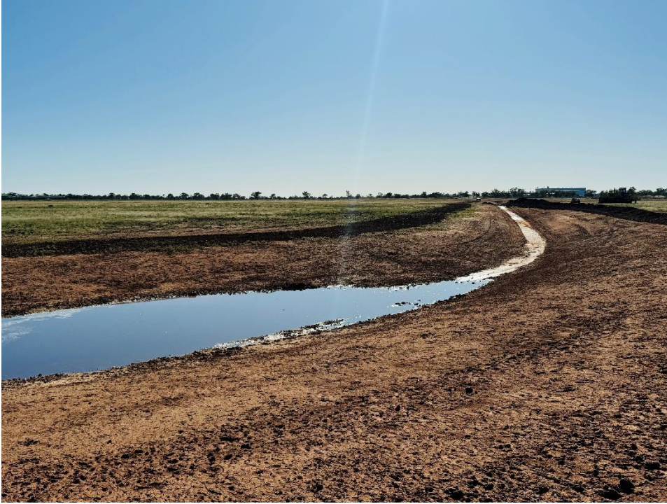
Figure 21: Tail-water Pond and Swale Drain
