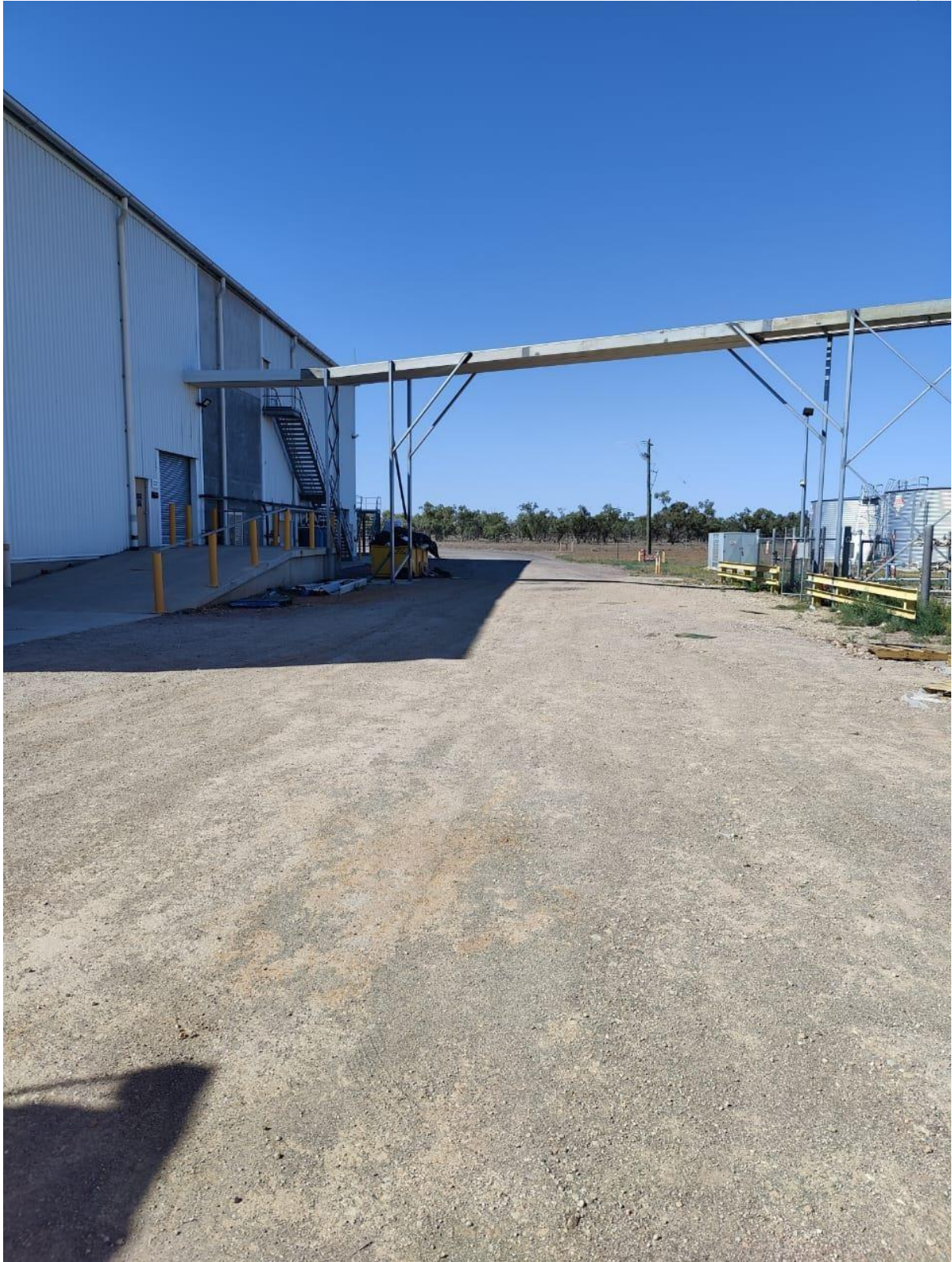
Figure 4: Backside road of the building
