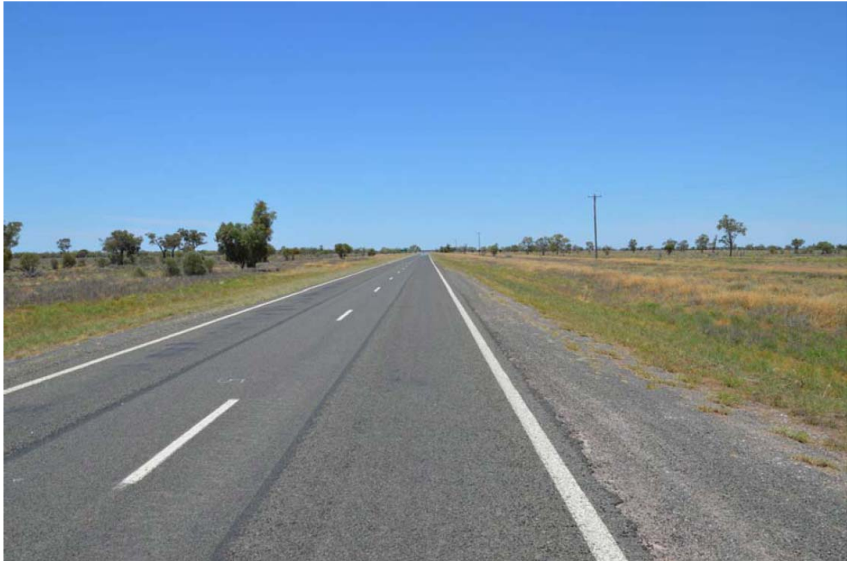
Photograph 2.1 Visibility on the Mitchell Highway at proposed site access looking south
