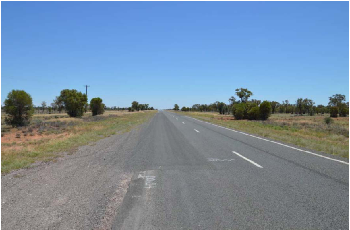
Photograph 2.2 Visibility on the Mitchell Highway at proposed site access looking north
