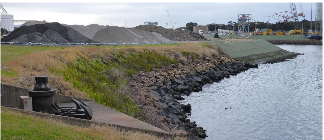
Figure 2-5 Southern Extent of Site 2 Near Discharge Point 3 (Looking North)
