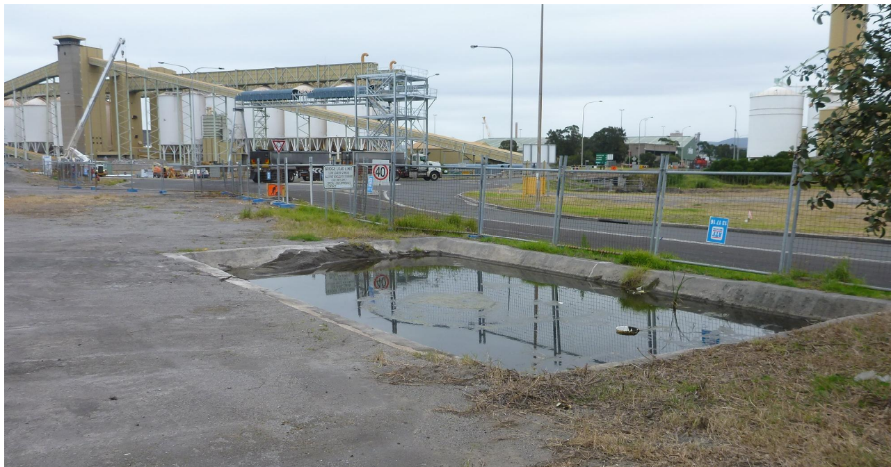
Figure 2-1 Existing Sediment Basin on Site 1 Adjacent to Tom Thumb Road (Looking West)
