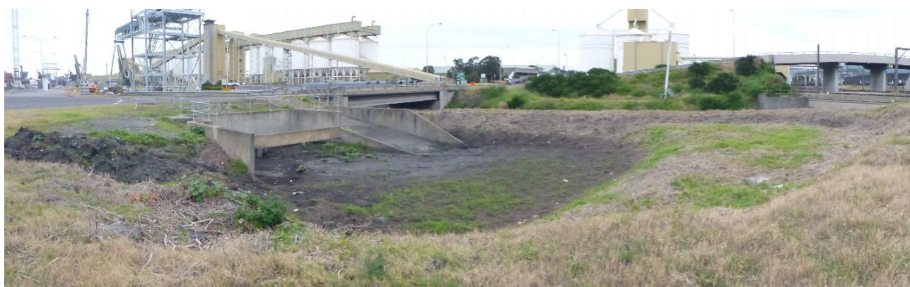
Figure 2-2 Existing Sediment Basin on Site 3 Adjacent to Gurungaty Waterway (Looking South-West)
