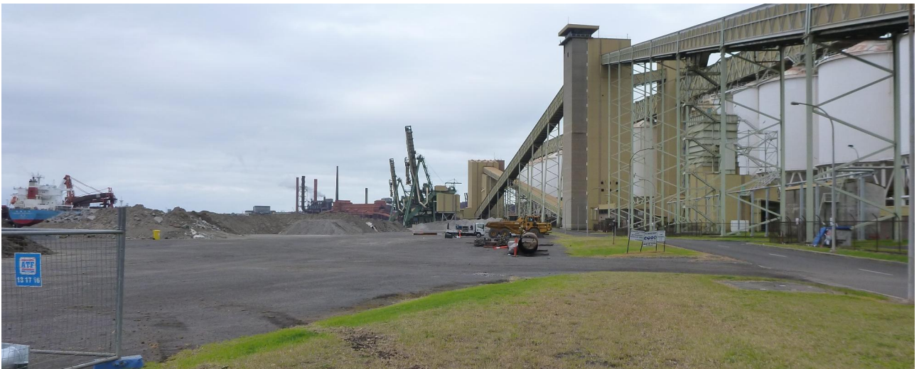
Figure 2-4 Site 2 Seen from the Intersection of Morton Way and Tom Thumb Road (Looking South)
