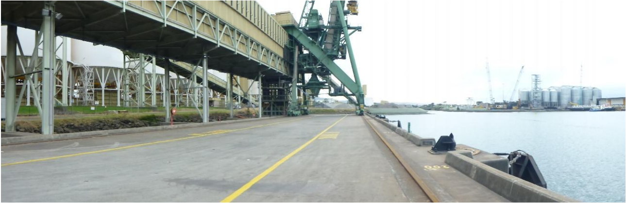
Figure 2-6 Berth 104 (Looking North)
