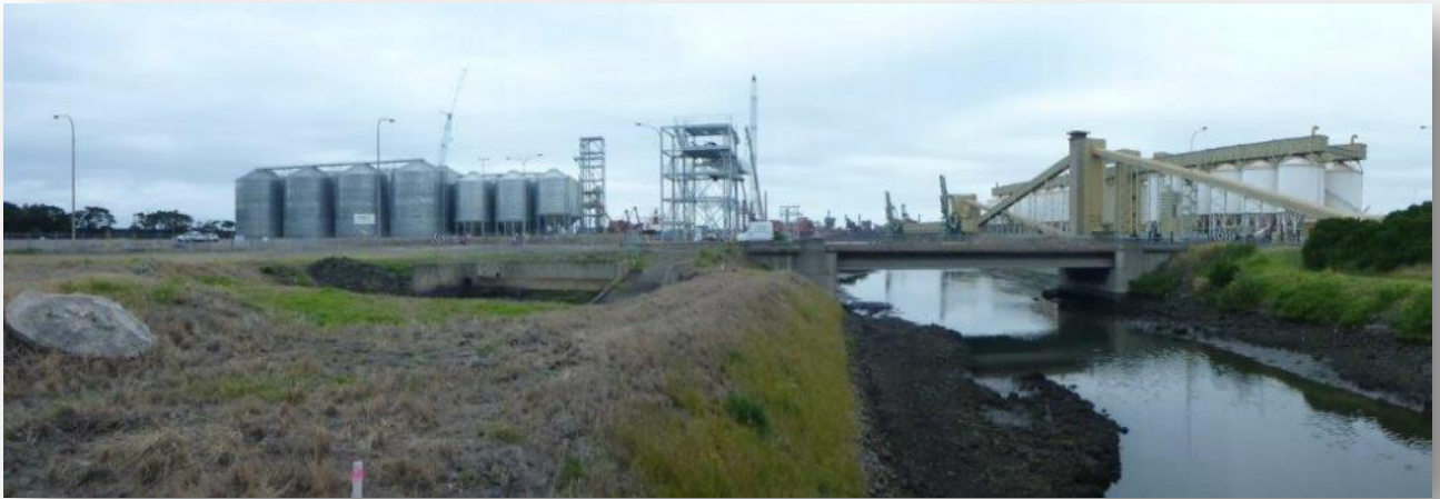
Figure 3-3 Panorama from waterway to the Inner Harbour including the GrainCorp Silos and new silos under construction (View Point 9)
