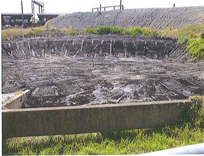
Plate 6. Allotment 6 facing north. The stormwater pit is in the foreground, and a large stockpile of gravel is present to the north.
