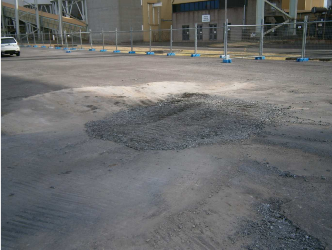
Photo 11: Test pit CTP01 (in Zone 1) after recompaction with backfill soils
