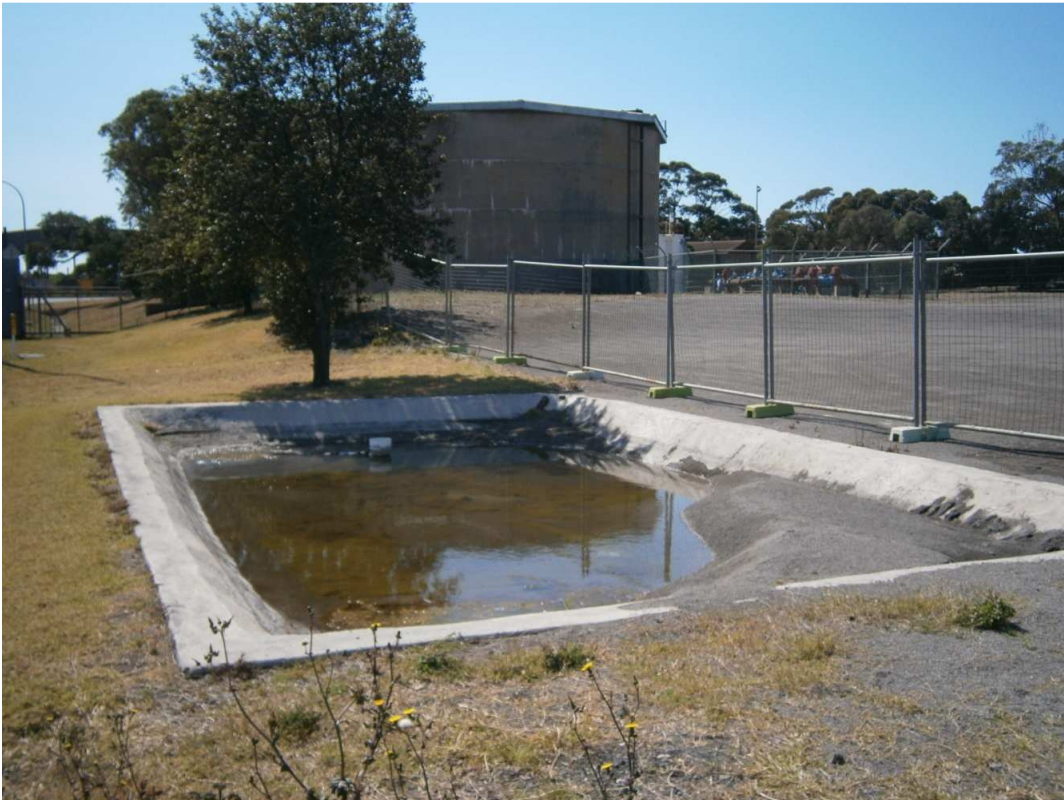
Photo 6: Concrete basin between Tom Thumb Road and southern area of Zone 2
