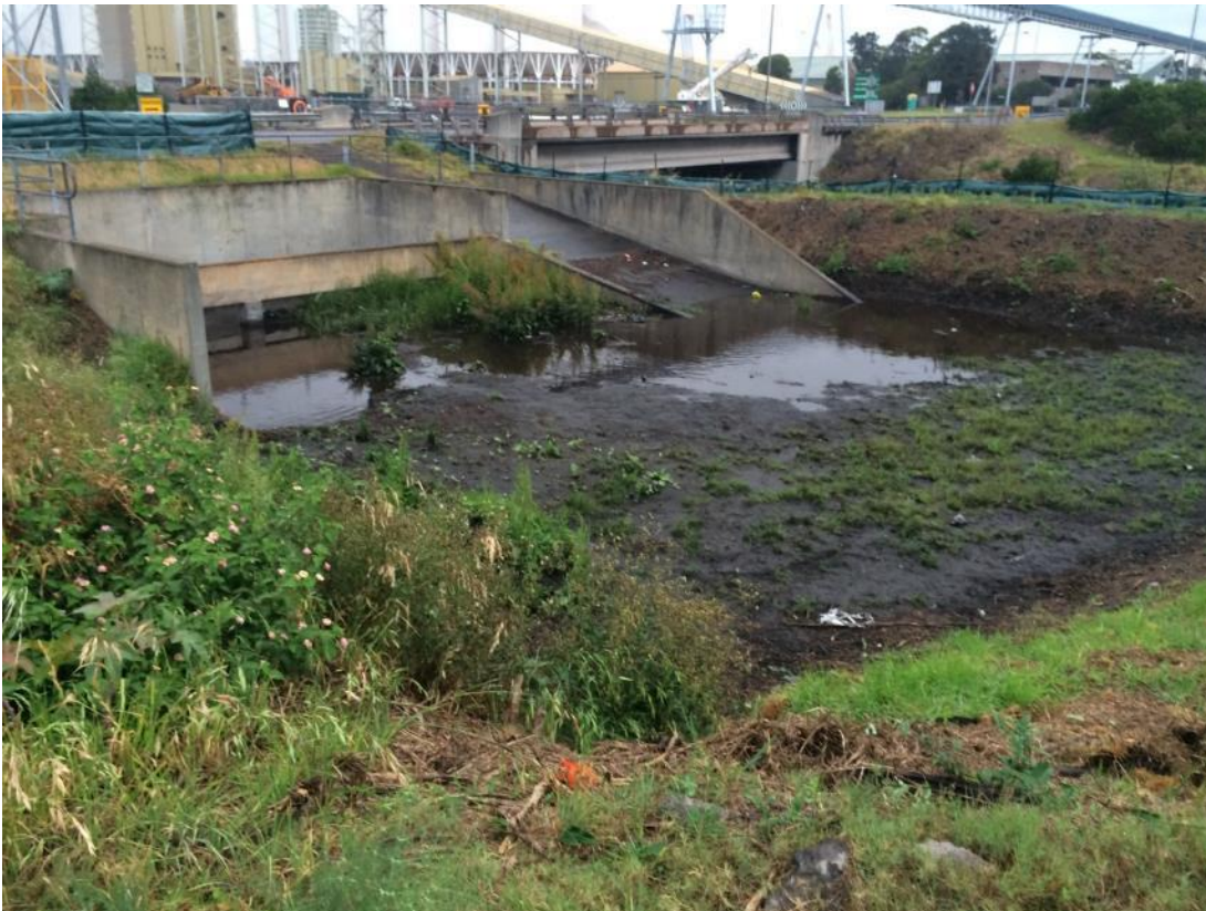
Photo 2.2: Stormwater detention basin on Site 3, within the study area.
