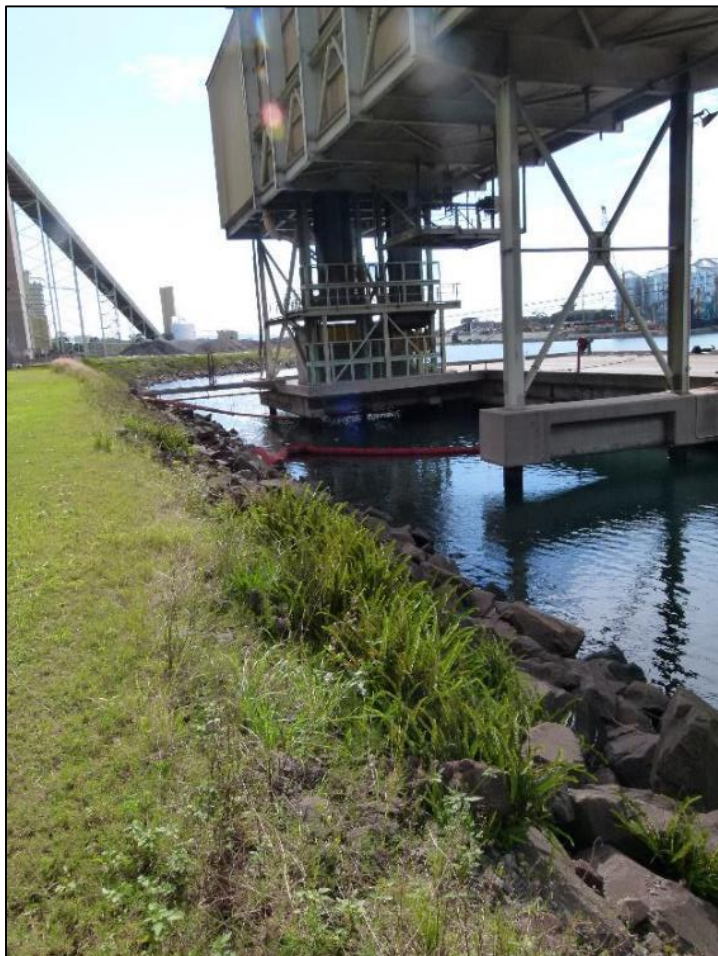
Figure 3-6 Breakwall at Site 2, colonised by Nephrolepis cordifolia * (Fishbone Fern) and Bidens pilosa * (Cobblers Pegs)
