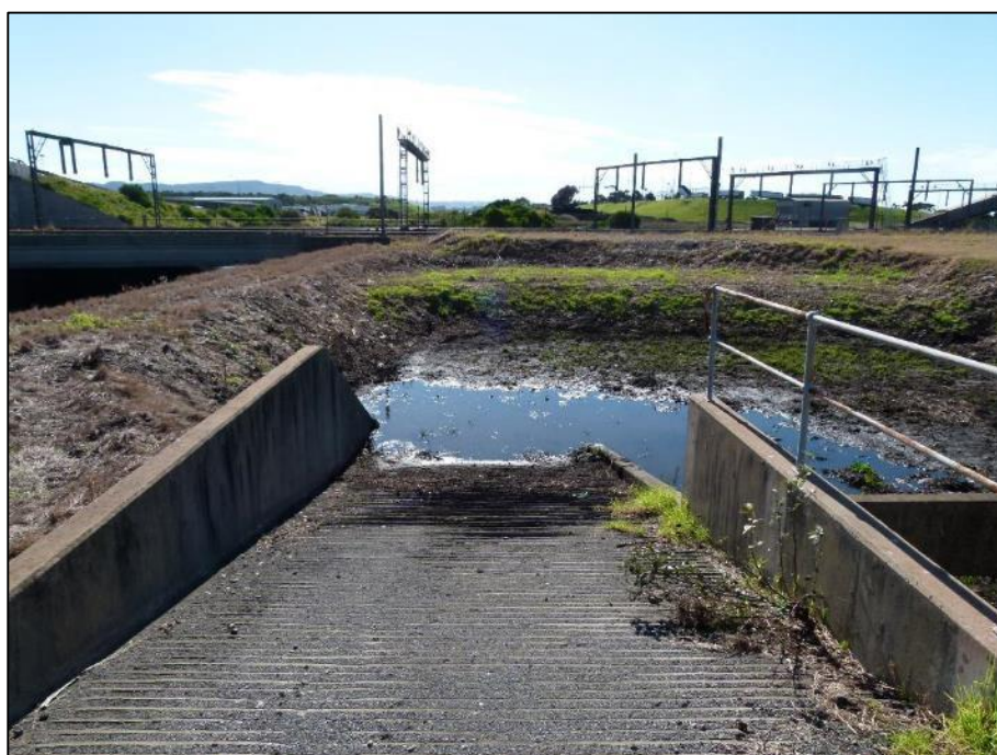
Figure 3-7 Stormwater Detention Basin at Site 3 with Sparse Grassy Groundcover
