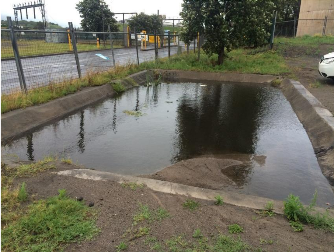
Photo 2.1: Stormwater detention basin on Site 1, within the study area.
