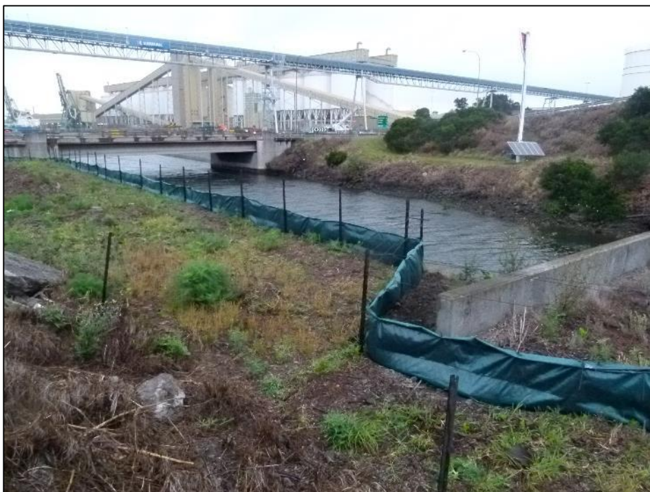
Figure 3-12 Gurungaty Waterway, looking south from Site 3. Temporary frog exclusion fencing can observed being erected along the waterway boundary
