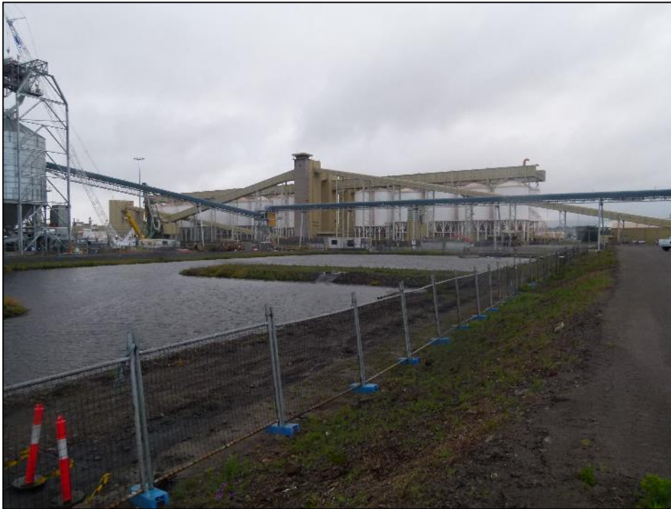
Figure 3-13 The Port Kembla Coal Terminal Settlement Ponds to the south of Site 1
