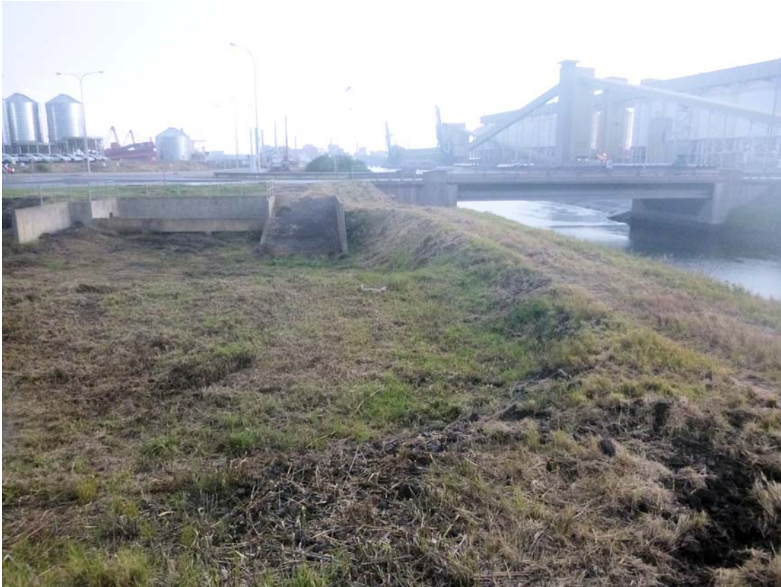
Figure 4 Storm water detention basin in Area 3
