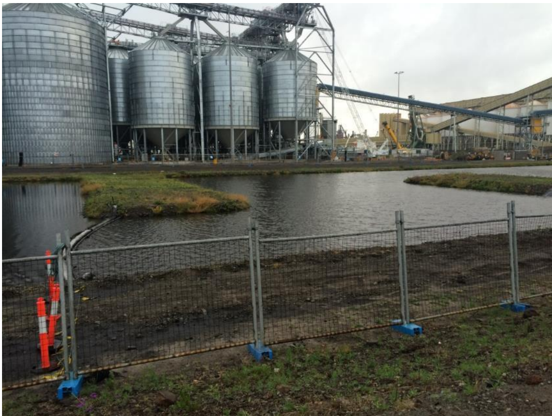
Photo 2.6: Large detention basin immediately to the south of the subject site (Site 1), potential breeding habitat which may encourage transitory individuals to pass through the subject site.
