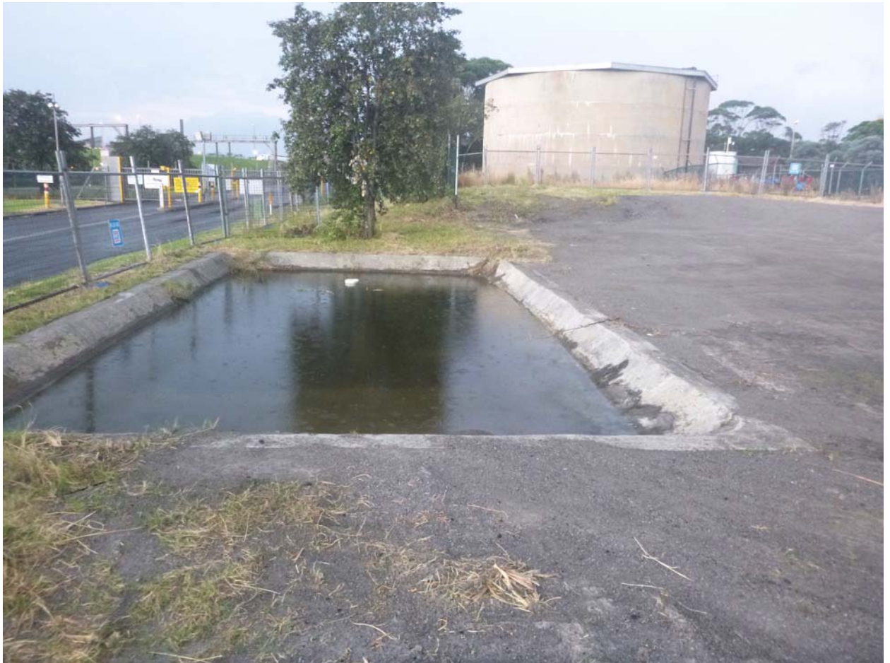
Figure 3 Storm Water sump in Area 1
