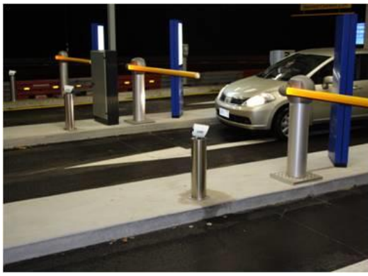
Figure 7.5: Car Park Exit Infrastructure
