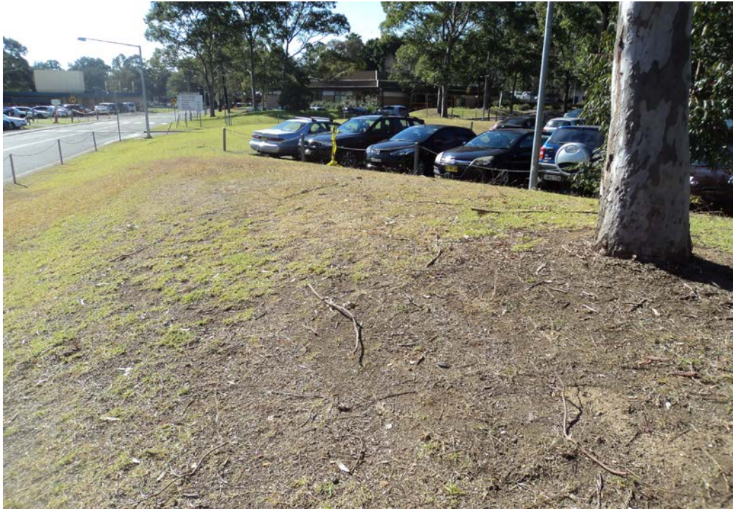
Photo 5 - Mounded soil in grassed area
