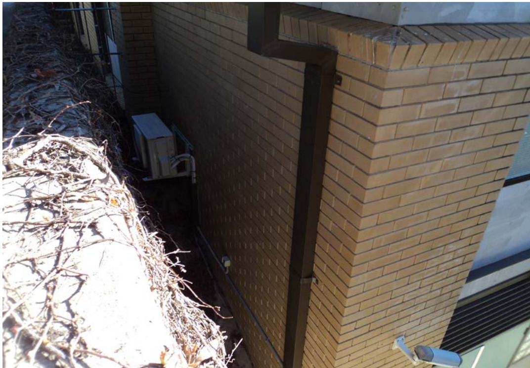
Photo 3 - Retaining wall next to office building
