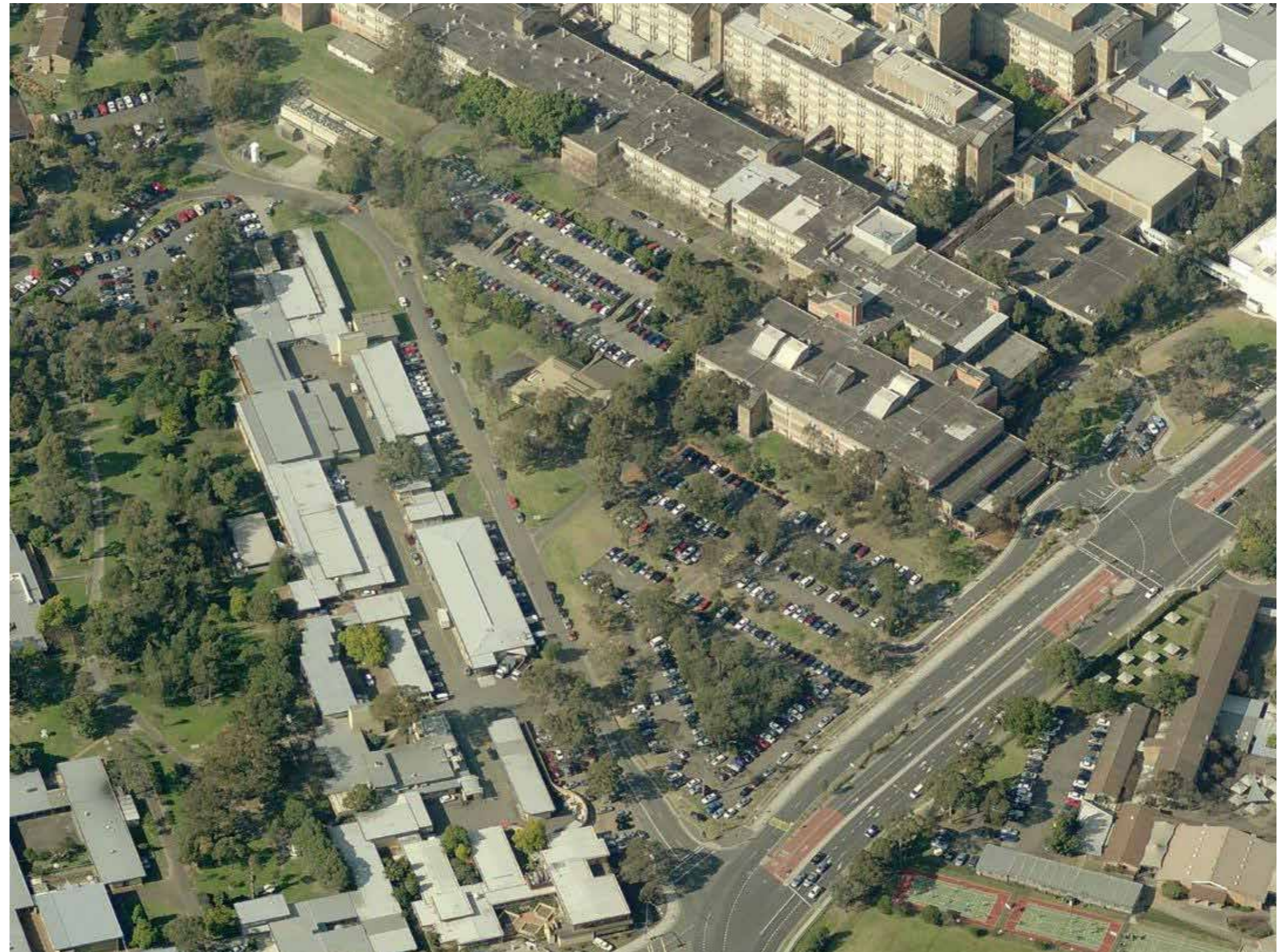
existing aerial view
