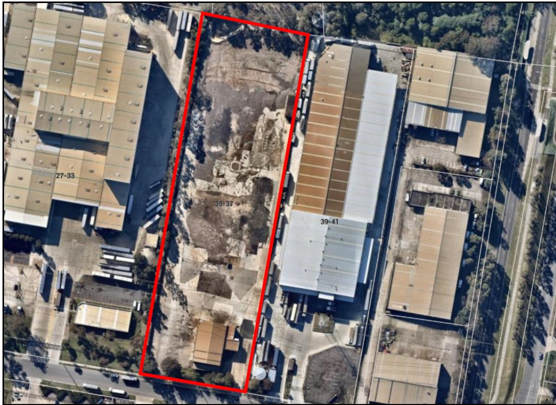
Figure 2: Aerial photograph showing the Site and the existing extraction operation on the Site.
