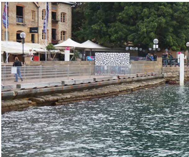
Fig. 25: Existing Heritage Sea Wall
