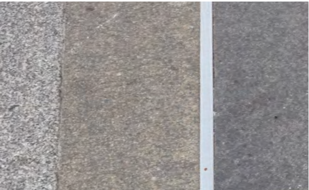
Fig. 24: Precedent - Range of Paver Types and Finishes and finishes at Customs House
