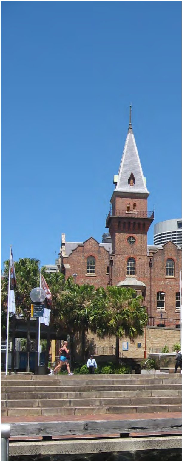
Fig. 19: Existing sandstone promenade steps
