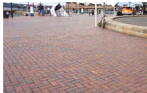
Fig. 5: Existing Campbell's Cove Promenade Paving
