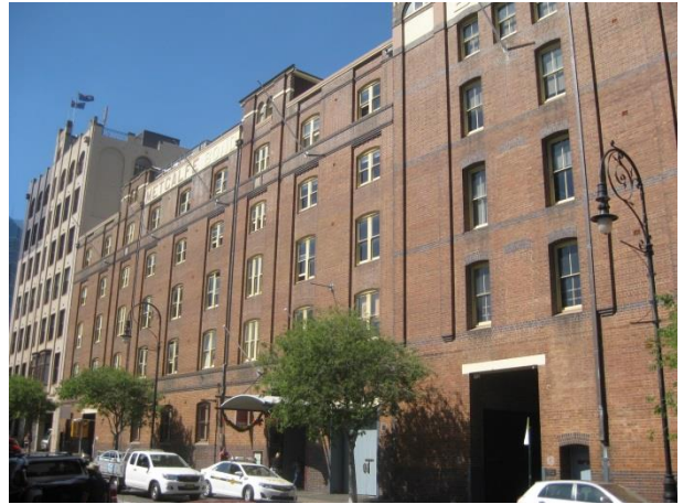
PICTURE 16 – METCALFE BOND STORES TO WEST OF CAMPBELL'S STORES
