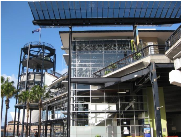
PICTURE 11 – OVERSEAS PASSENGER TERMINAL
