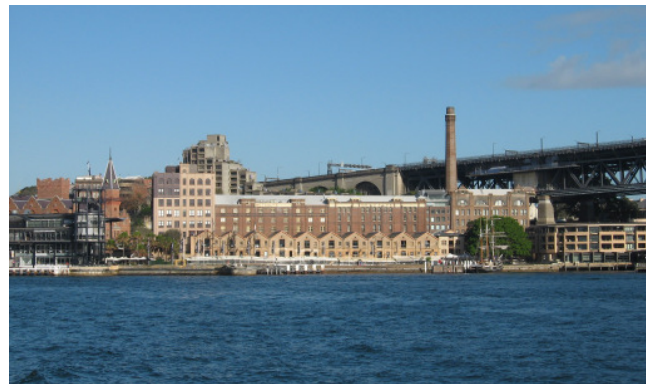
Figure 3.2 Campbells Cove from the harbour with the gable fronted facade of Campbells Stores that provides a backdrop to the promenade
