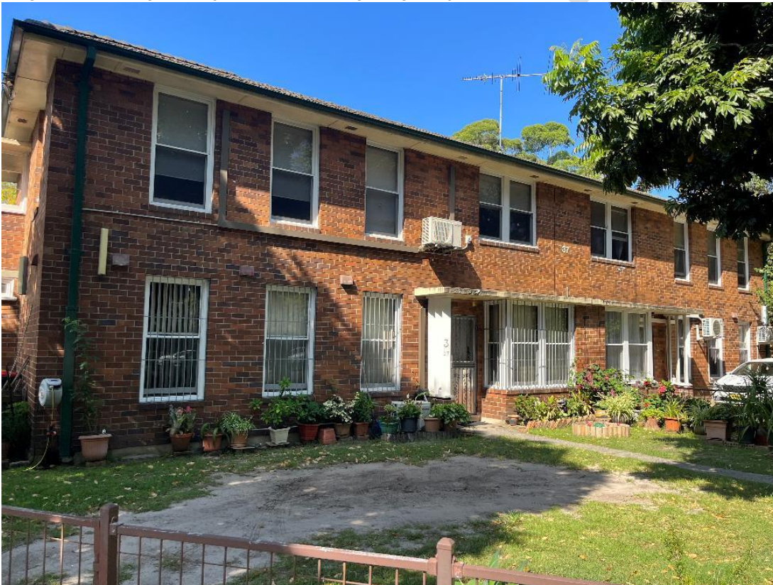
Image 0.1 View of high density residential building along Henry Kendall Crescent, facing north east
