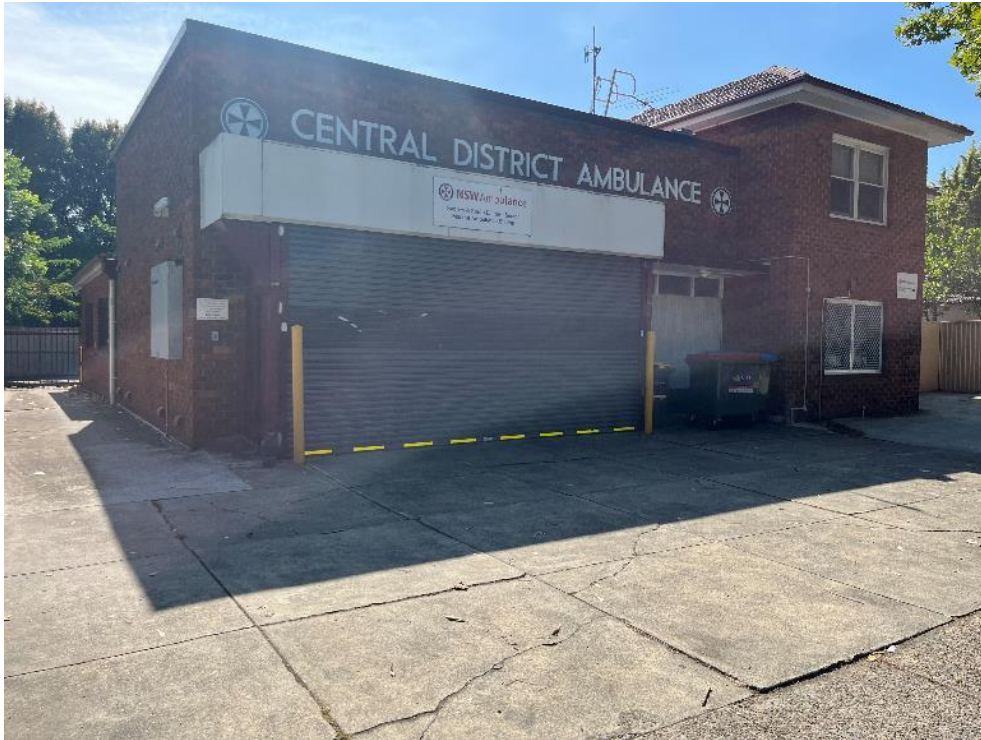
Image 0.2 View of operational NSW Ambulance Station along Botany Road, facing west
