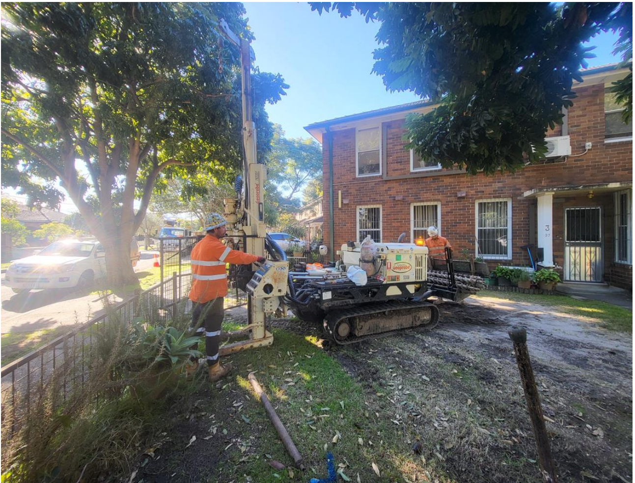
Photo 1 – Drilling set-up near CPT01
