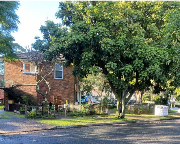
Picture 3 View of the site facing south on Henry Kendall Crescent
