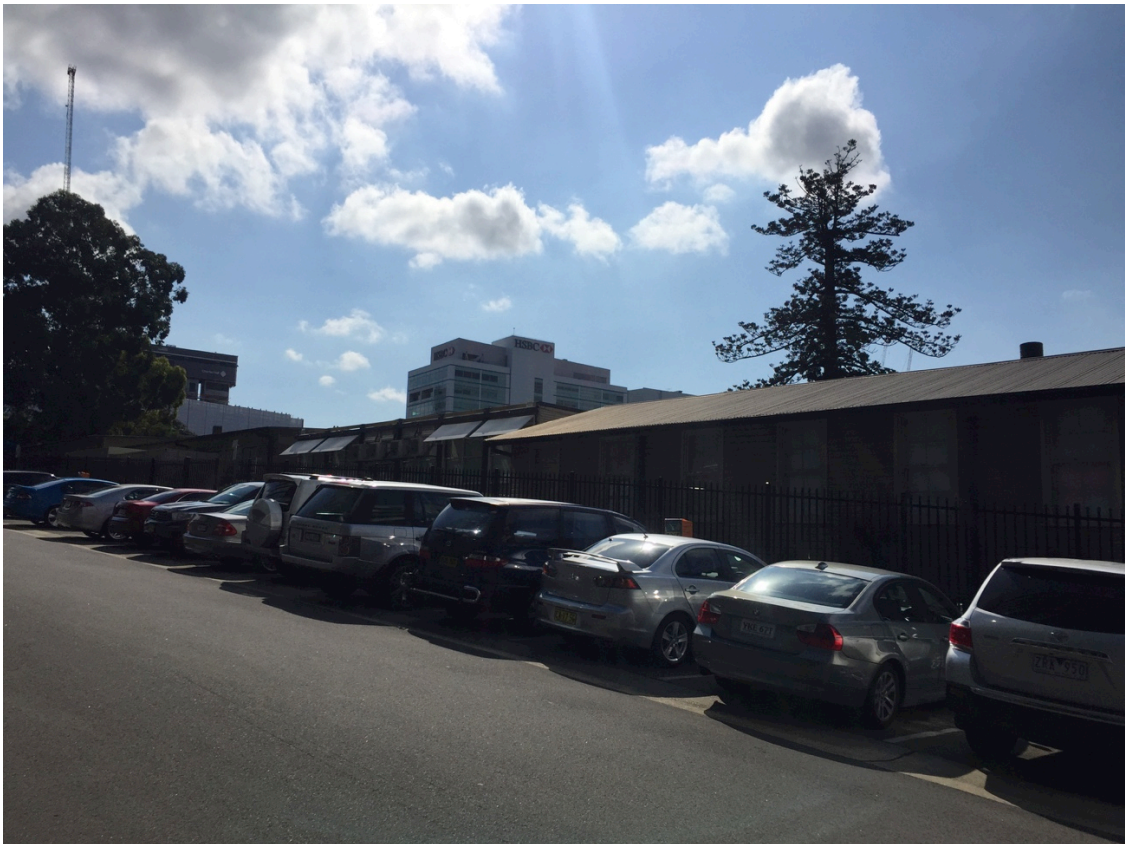
Figure 6 Little Street and southern elevation of the PPS site Source: Mecone
