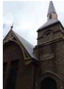
3. Old School House Building
