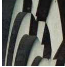
Insitu concrete amphitheatre
