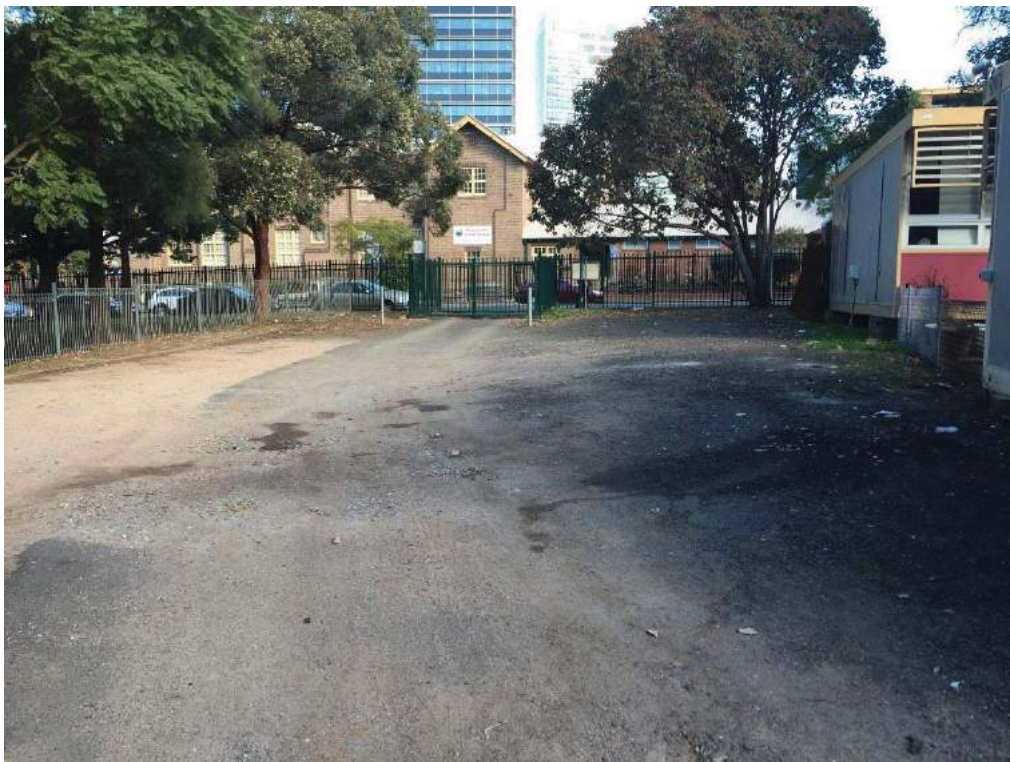
Photograph 1: Driveway and car park of northern portion of the site, looking south. Location of boreholes BH4, BH5 and BH6.
