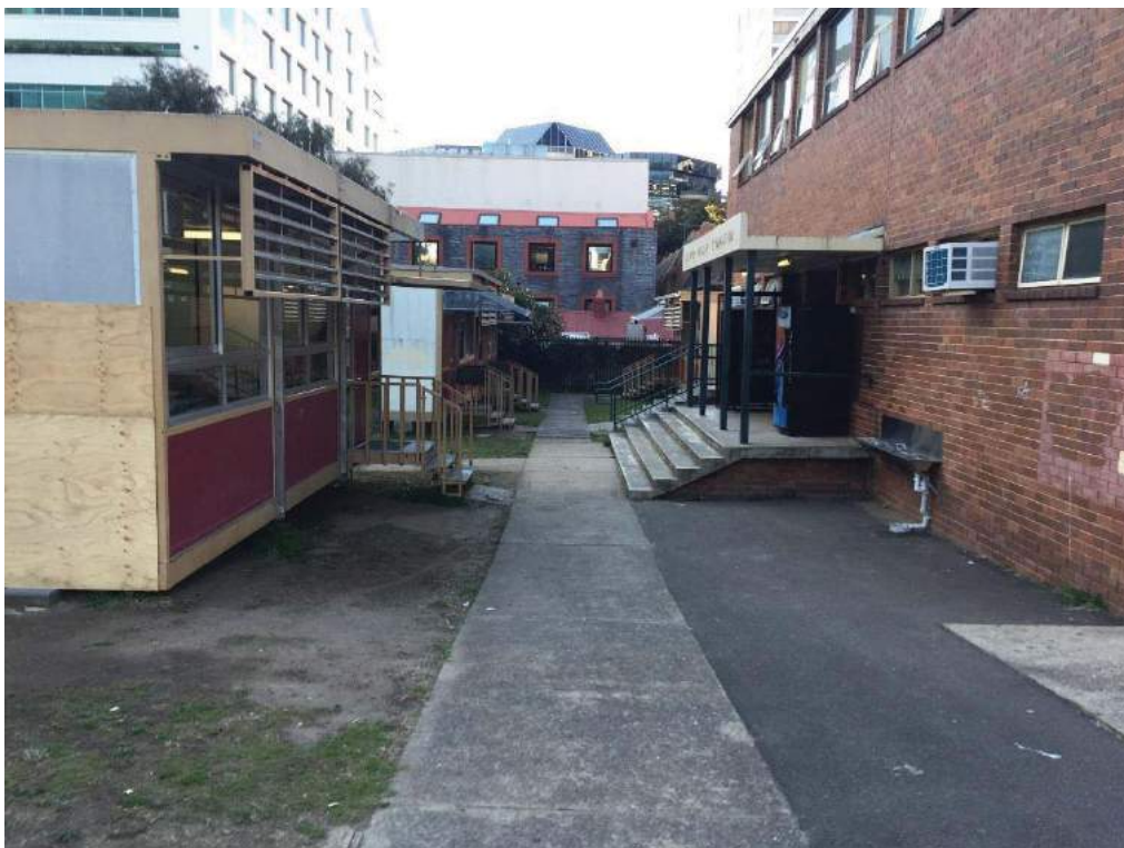
Photograph 2: Western side of school hall and demountable buildings, looking north.
