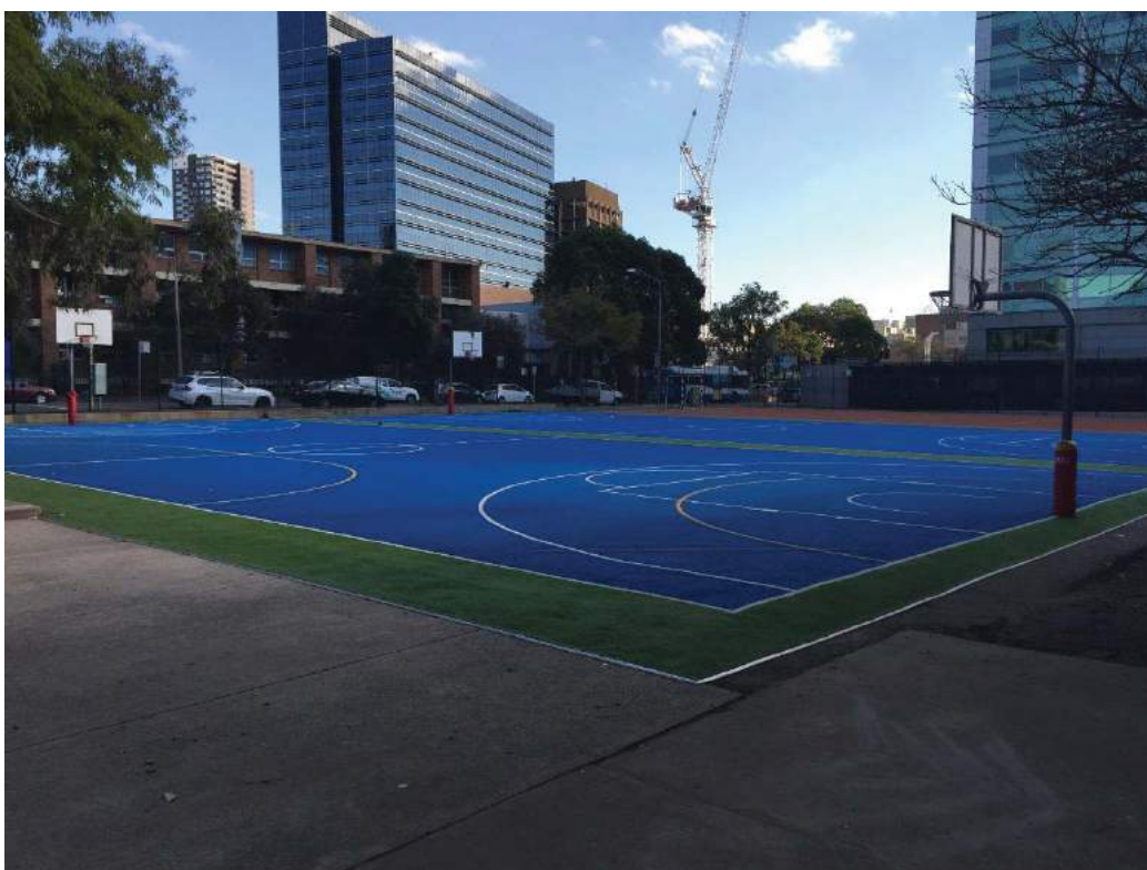
Photograph 4: Sports Courts at Arthur Phillip High School, looking south-west. Inaccessible area for borehole drilling.
