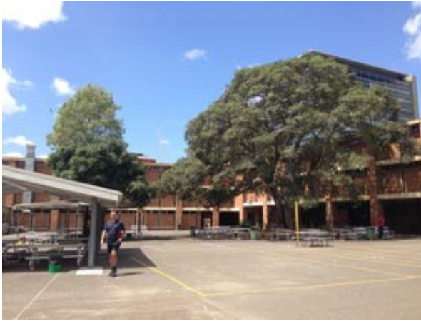
Figure 3.1 View looking southeast showing the central courtyard of APHS. (GML 2016)
