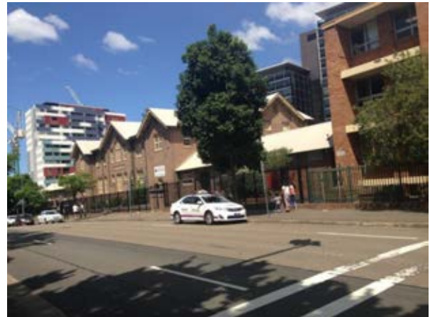
Figure 3.4 View looking southeast showing the row of the 1923 PPS heritage buildings along the Macquarie Street frontage. The drop towards Charles Street in the east is prominent. (GML 2016)
