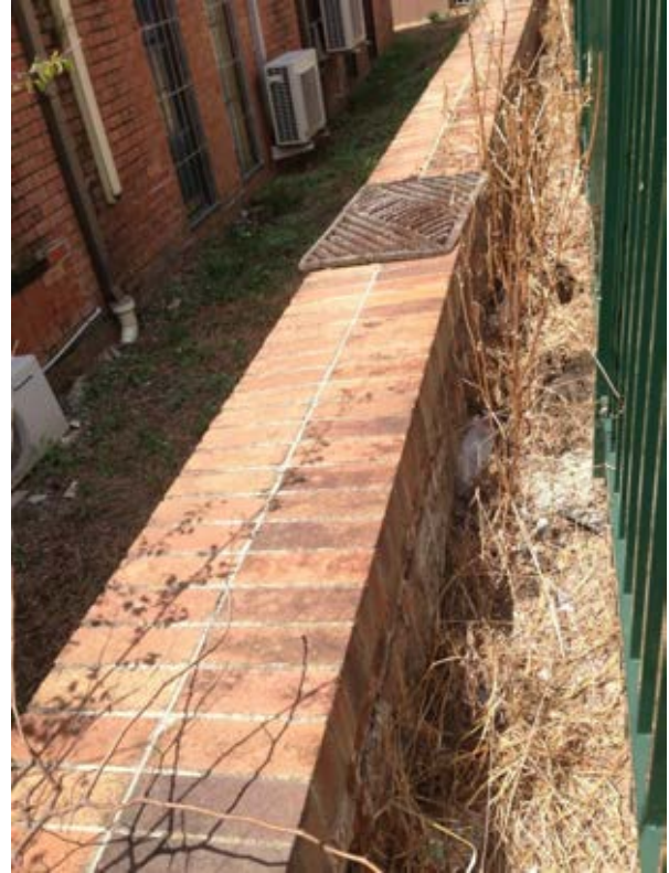
Figure 3.10 The middle section of the heritage brick wall is only a few courses high and capped with modern bricks. (GML 2016)
