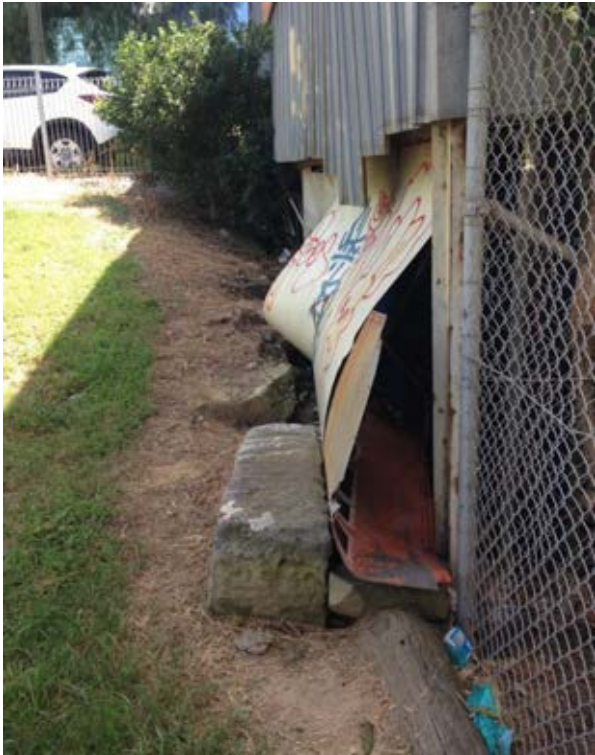
Figure 3.11 Dislodged sandstone foundation stones are all that is left of the heritage convict wall in the east end of its original length. (GML 2016)
