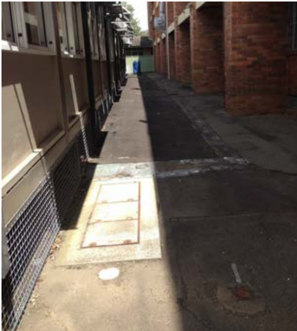
Figure 3.3 View looking south showing the location of services in the passageway between the APHS and PPS sites. (GML 2016)
