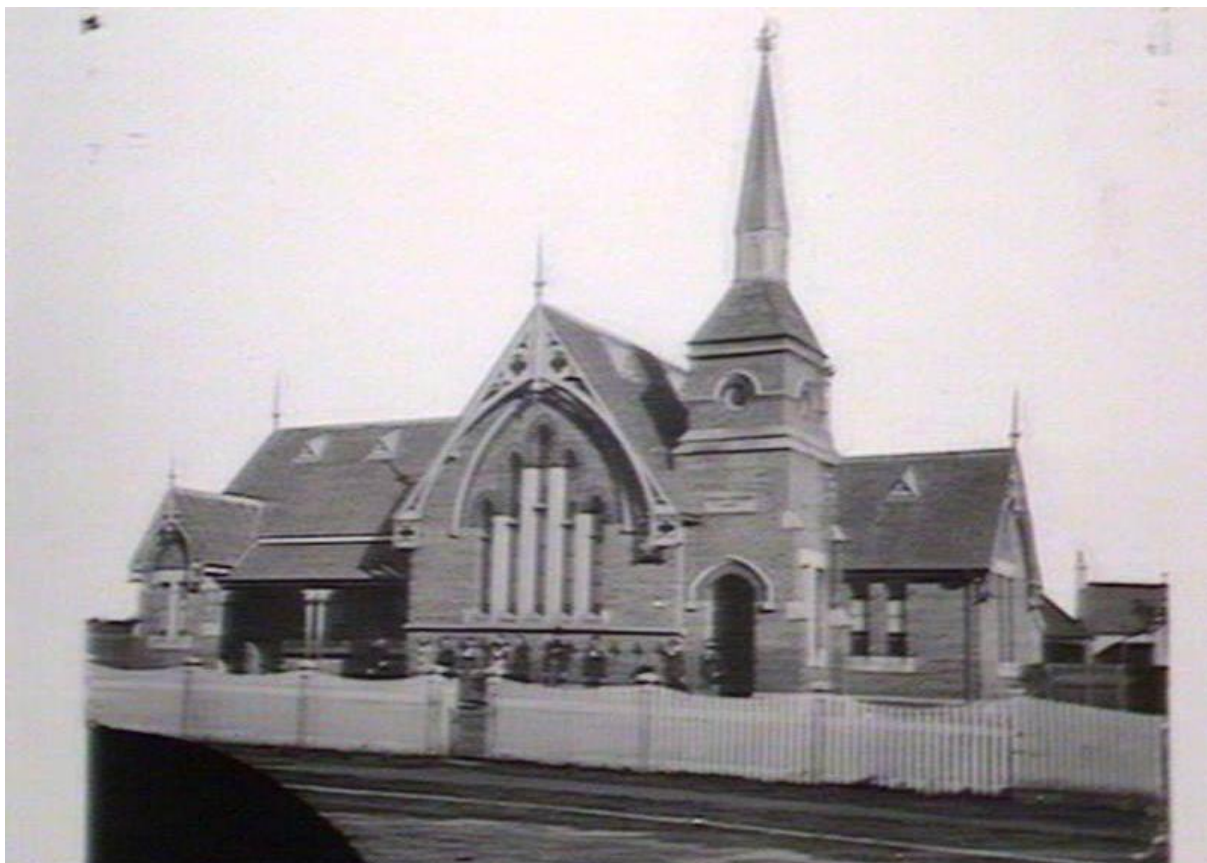
Figure 2.15 Original school building, built in 1875, now part of Arthur Phillip High School. Date unknown. (Source: Public School, Parramatta, SLNSW, Digital Order Number d1_06150)
