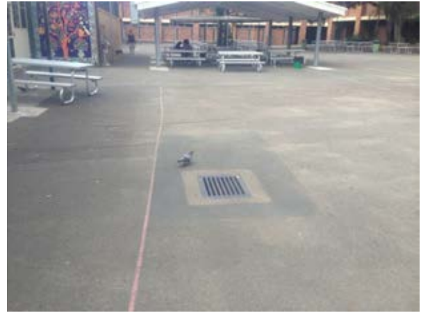
Figure 3.2 An outlet of a stormwater drain which runs across the central courtyard in a north-south direction and exists the site through the Macquarie Street side gate. (GML 2016)
