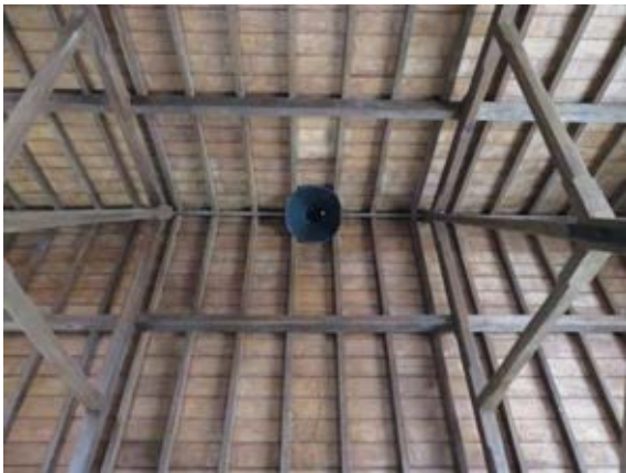
Figure 3.11 Ceiling of the eastern school room showing a conical ventilator.
