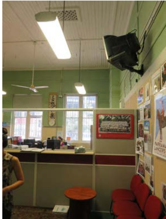
Figure 3.24 The southern school room in the 1890s addition (now office) showing the chimney breast in the northwest corner.
