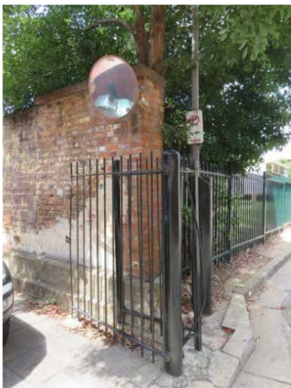
Figure 3.61 The western end of the convict barracks wall showing a section of early sandstock brickwork. A concrete kerb has been built along the side of the sandstone plinth. A new brick capping has been added to the wall.
