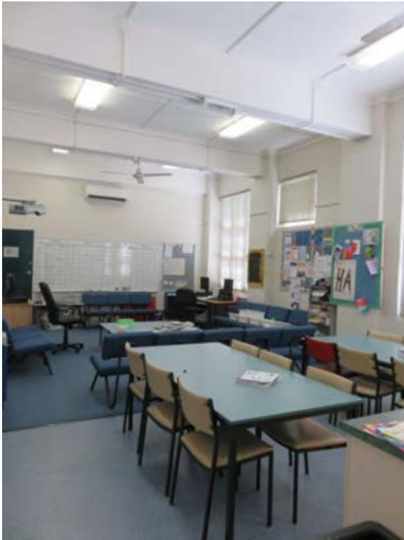
Figure 3.45 The northern space on the ground floor showing deep beams supporting the floor above.
