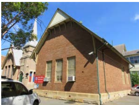
Figure 3.5 North elevation of the 1890s addition. Note the fanlights above the windows have been removed.
