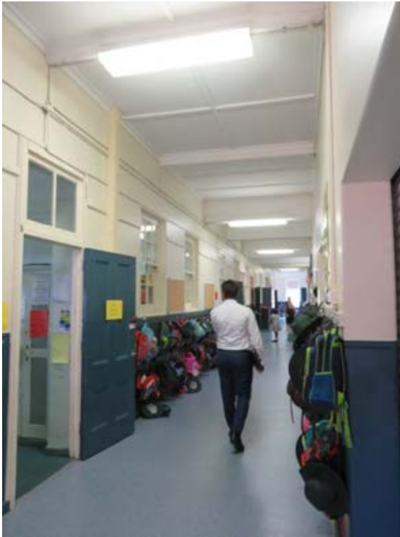
Figure 3.39 The ground floor corridor looking west, showing windows and doors to the southern classrooms and exposed beams supporting the floor above.
