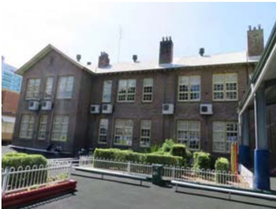
Figure 3.29 South elevation of the 1923 school building.
