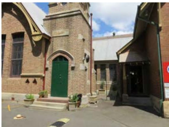
Figure 3.7 View of small entrance porch to the 1890s addition (right) and into the small northern courtyard between the addition and the original building.
