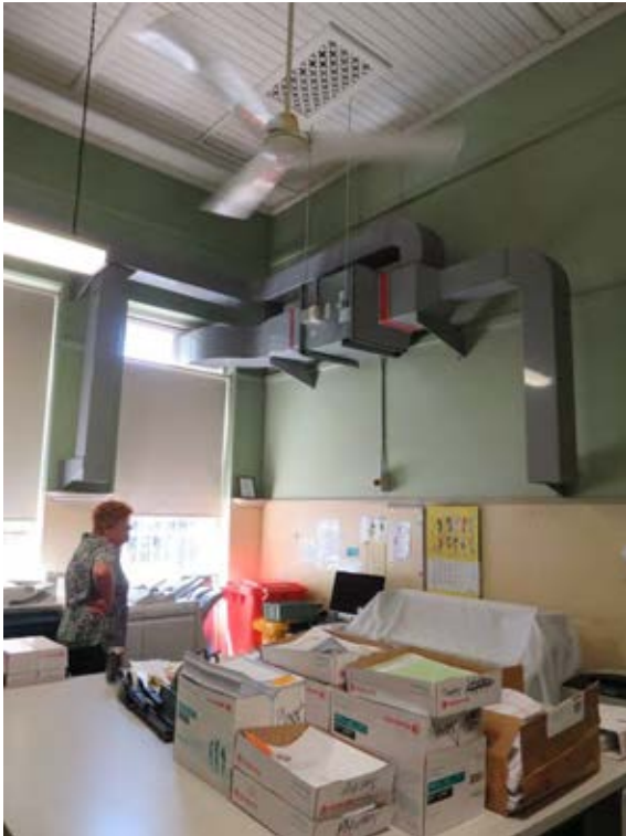
Figure 3.23 The northern school room in the 1890s addition with air conditioning ductwork mounted on the late twentieth century partition wall dividing school room into two spaces.
