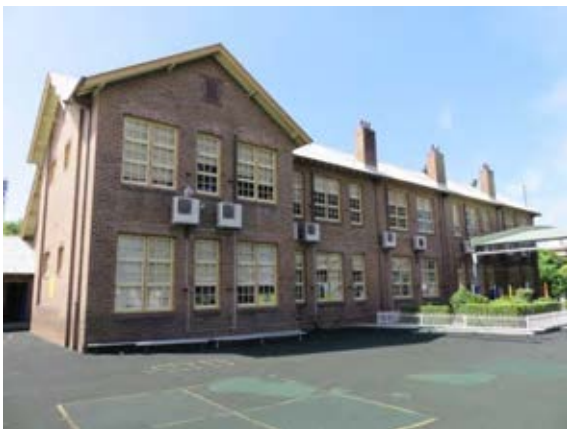
Figure 3.31 South elevation of the 1923 school building.
