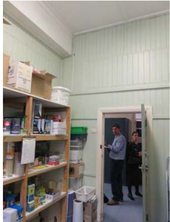
Figure 3.46 An early vertical boarded partition showing high level openings boarded up.
