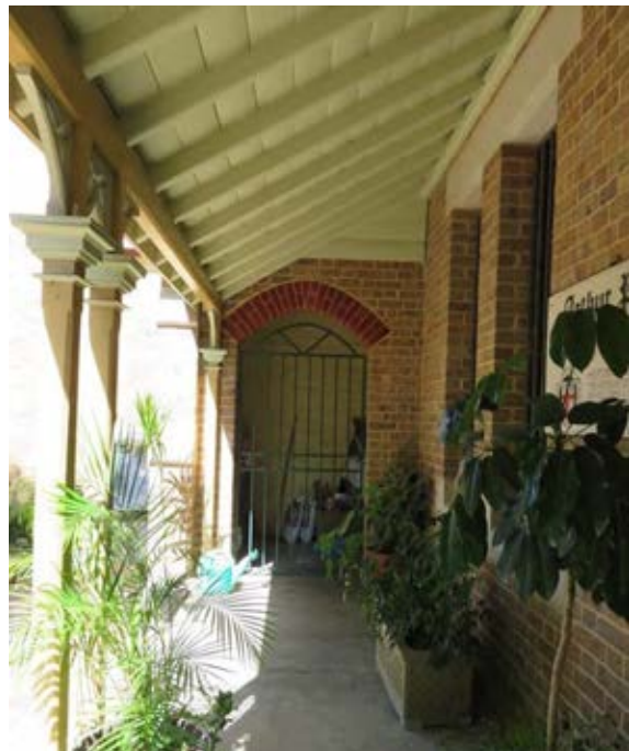
Figure 3.3 View along the front verandah towards the northeast entrance porch.
