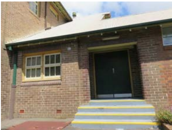
Figure 3.35 North elevation of the western entrance porch.
