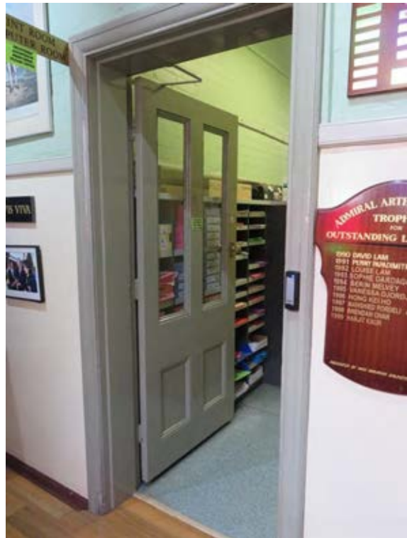
Figure 3.22 The original panel door to school room in the 1890s addition with the upper panels replaced in glass.
