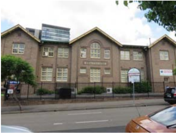
Figure 3.27 North elevation of the 1923 school building showing contrasting brick trim.
