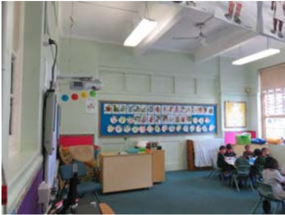
Figure 3.41 The southern classroom on ground floor showing folding doors boarded joinery in opening between classrooms. Exposed beams supporting floor above.
