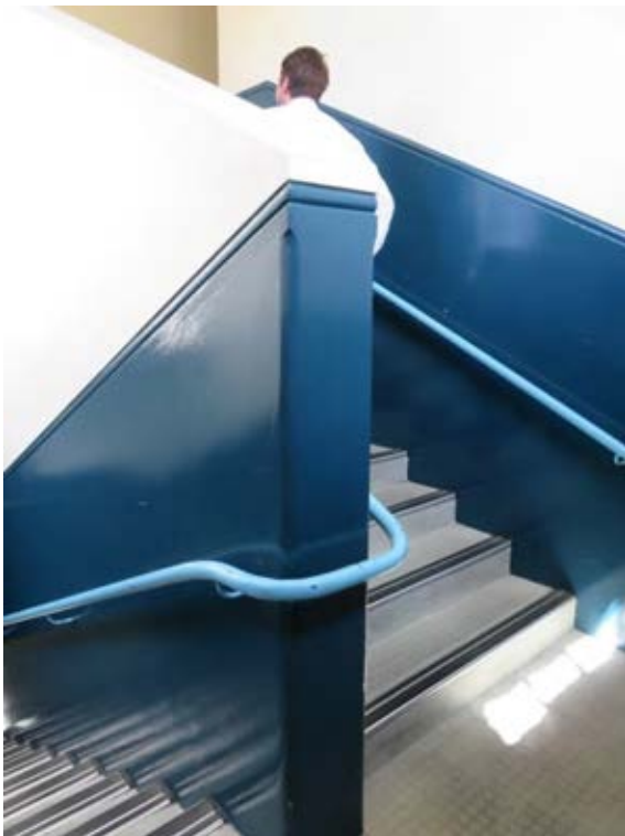
Figure 3.47 A concrete stair with a run dado in the wall.
