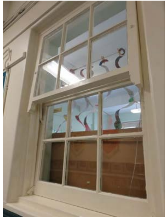
Figure 3.40 Typical window to the corridor showing the original brackets.
