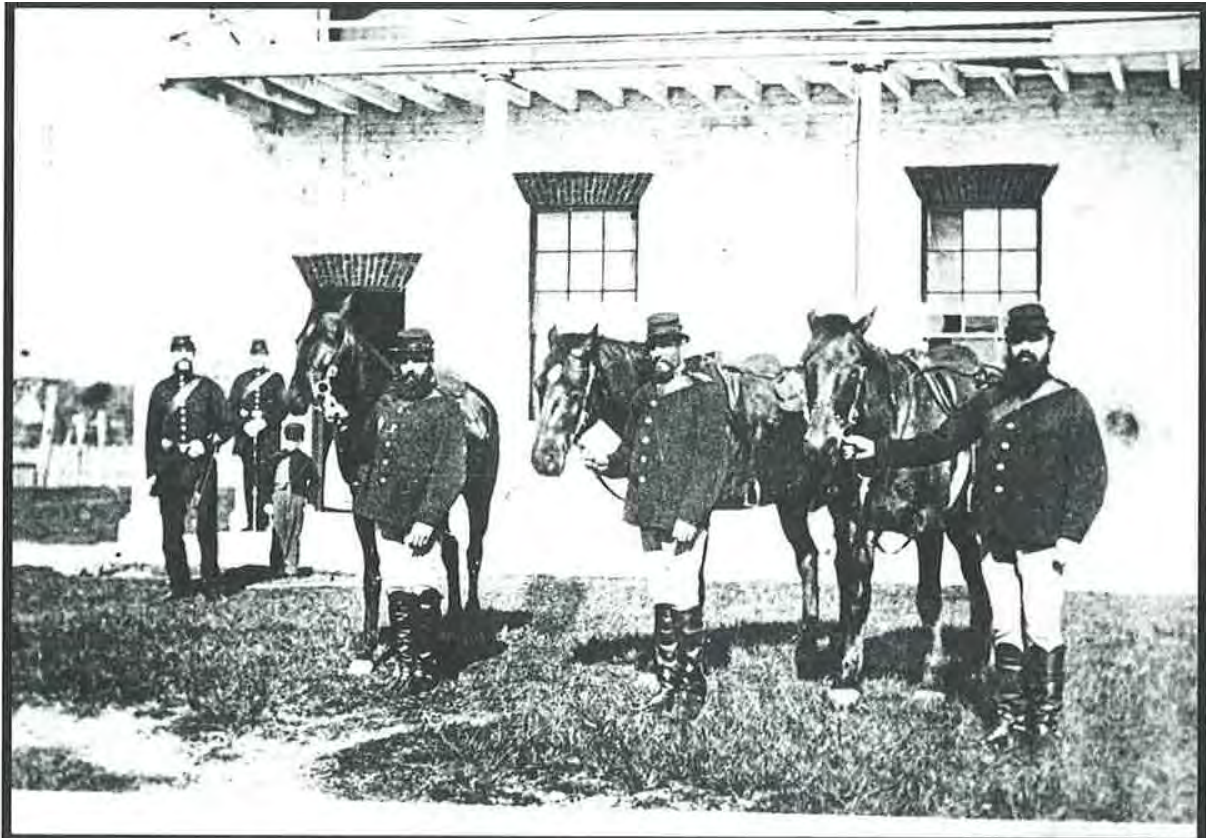
Figure 2.11 Police Barracks, now the Lancer Barracks, c1870. (Source: S & K Brown, Parramatta: a town caught in time , Sydney, Hale & Iremonger, 1995.)
