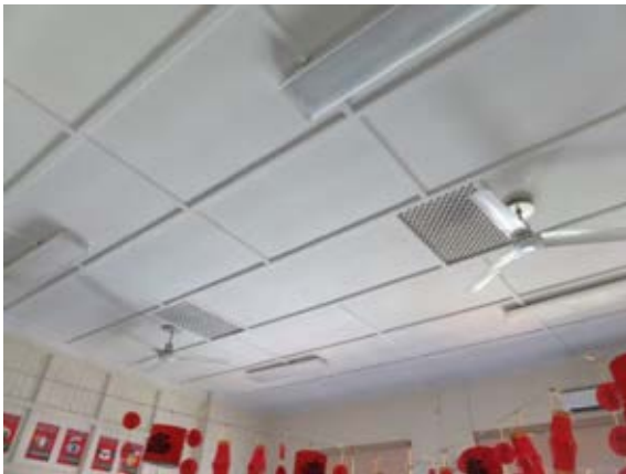
Figure 3.51 A battened ceiling on the first floor showing rectangular ventilation panels.
