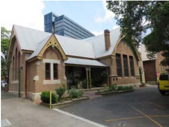
Figure 3.1 North elevation of the 1875 school building with a small entrance porch at the northeast corner.
