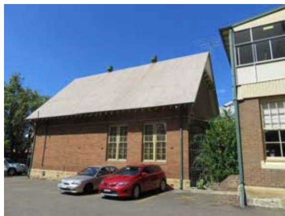
Figure 3.6 West elevation of the 1890s addition. Note the fanlights above the windows have been removed.
