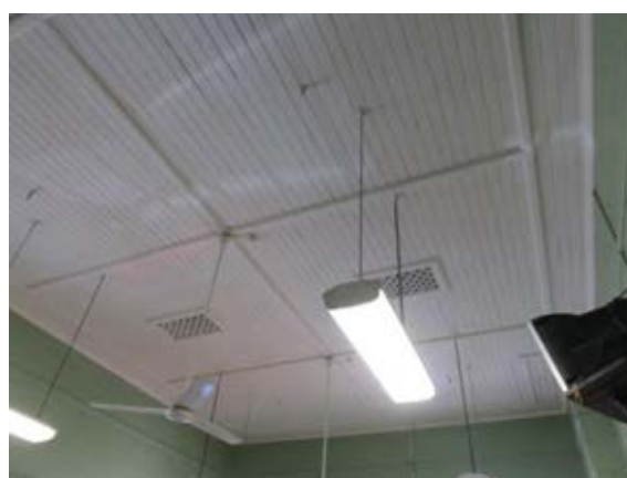
Figure 3.20 Boarded ceiling with battens and rectangular ceiling ventilation panels in the southern school room of the 1890s addition.
