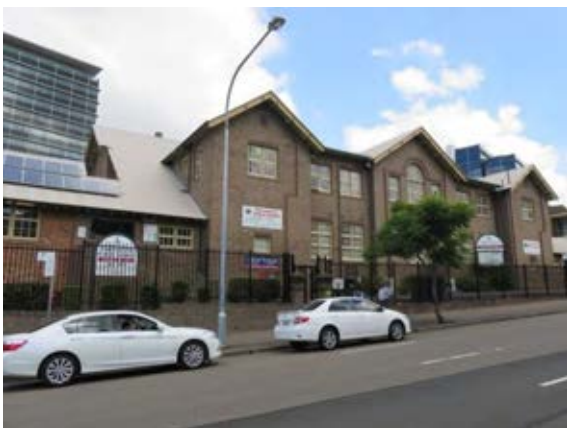
Figure 3.25 View of the 1923 school building along Macquarie Street from the northeast.
