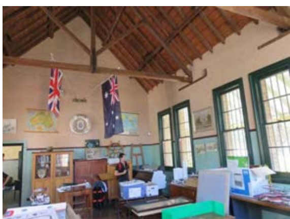
Figure 3.9 Eastern school room looking west, showing exposed trusses and rafters to the ceiling, the rendered dado around walls and original windows.
