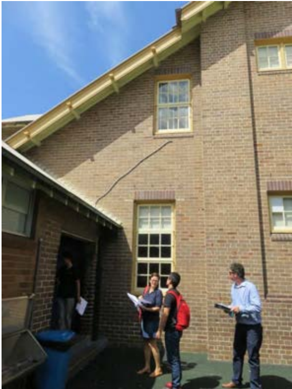
Figure 3.33 West elevation of the 1923 school building showing the western entrance porch.
