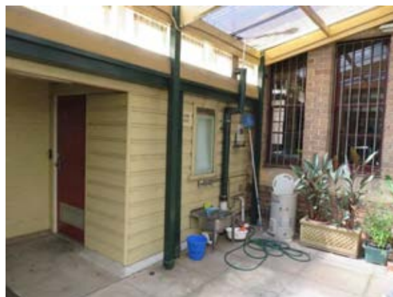
Figure 3.8 Weatherboard WC on the rear verandah.
