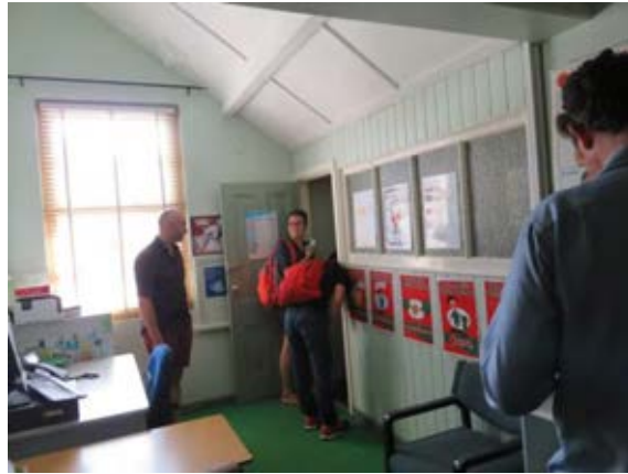
Figure 3.50 An early boarded and glazed partition enclosing a small space under raked ceiling on the first floor.
