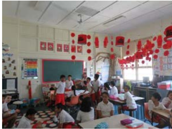
Figure 3.42 The southern classroom on the first floor showing folding doors, boarded joinery in the opening between classrooms and rectangular ventilation panels in the ceiling.
