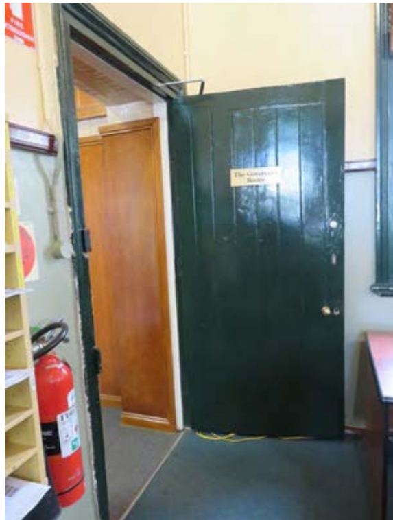
Figure 3.14 The original framed and sheeted door and architraves in the southern wall of the central school room.
