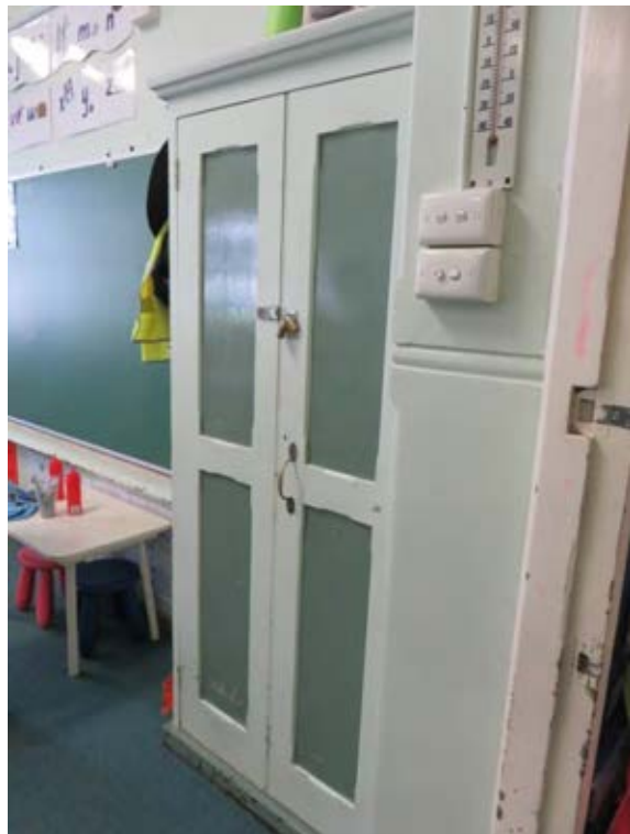
Figure 3.44 An early cupboard in the classroom. Note the moulded dado line run in the wall render.
