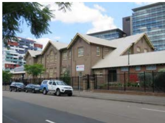
Figure 3.26 View of the 1923 school building along Macquarie Street from the northwest.
