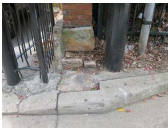
Figure 3.62 The western end of the convict barracks wall showing the sandstone blockwork to the base of the wall.
