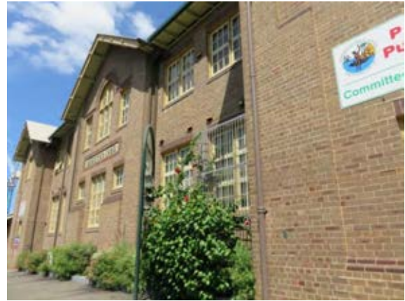
Figure 3.28 View showing the articulation of the north façade.
