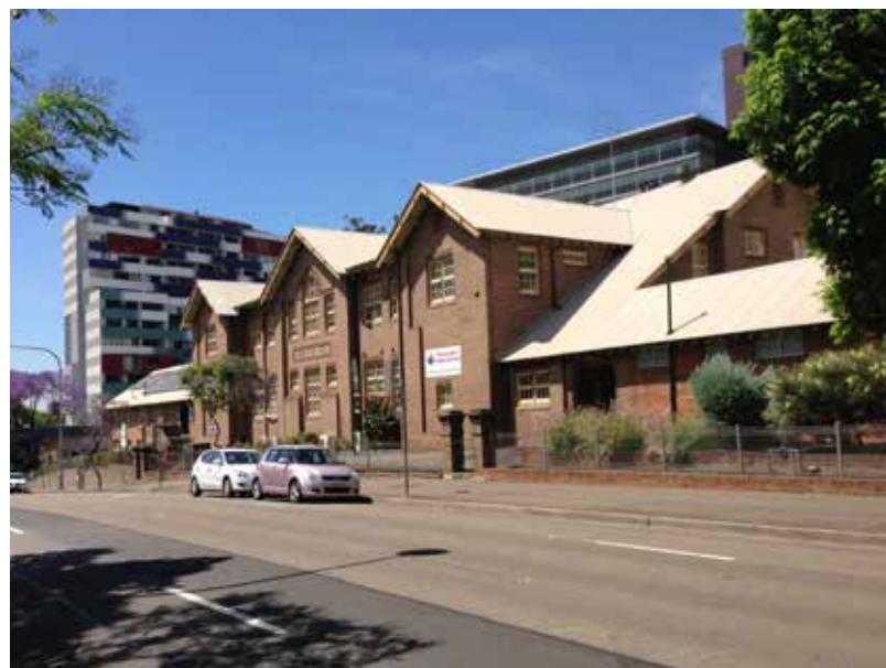
Parramatta Public School - View looking south-east along Macquarie Street
