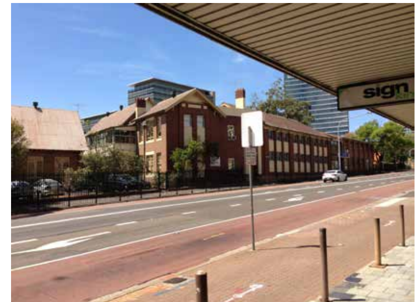
View from opposite north-west corner
