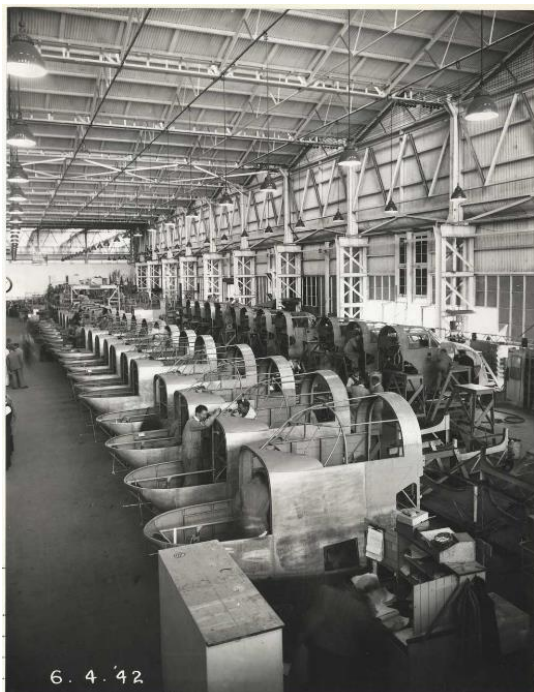
Figure 10: Construction of Beaufort Bombers undertaken at Chullora Rail Workshops during WWII
