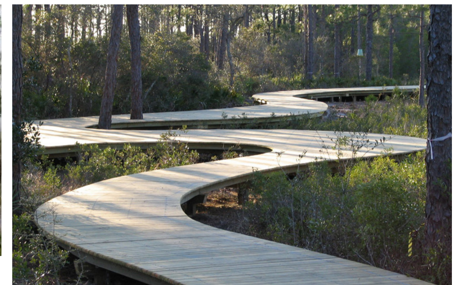
Slightly Raised walkways
