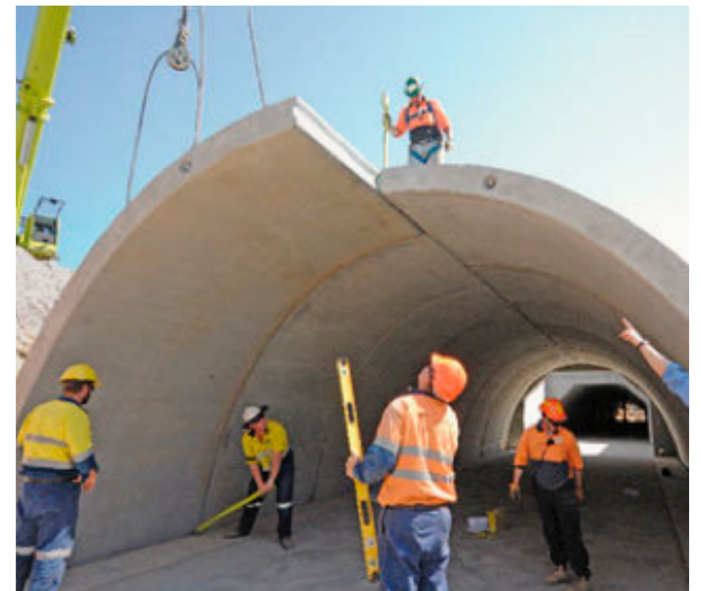
Construction of Pre Fabricated Concrete Panels
