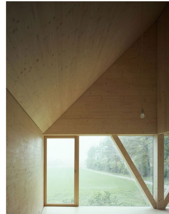
Cross Laminated Timber Panels
