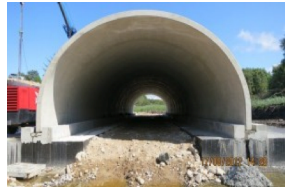
Construction of Pre Fabricated Concrete Panels
