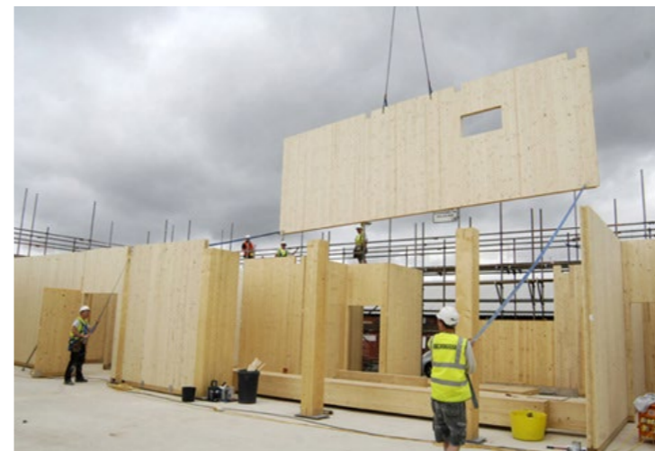
Cross Laminated Timber Panel building under construction
