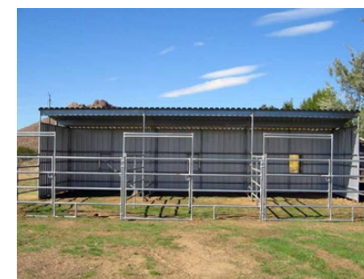
Service Yard Weather Shelters Enclosures and Building Form
