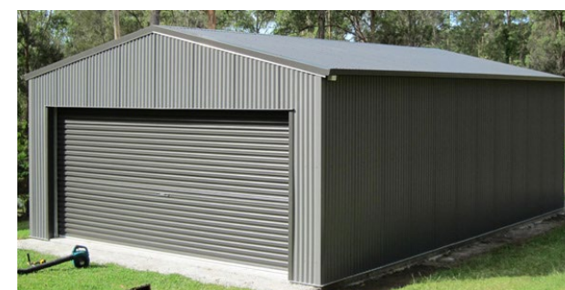
Works Depot Shed and Storage Bays for soil etc.
