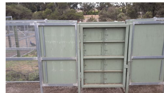
Giraffe Shelter and Gate
