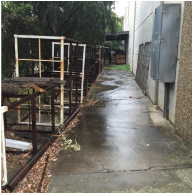
Photo 5.1.10 Concrete hardstand external to building
