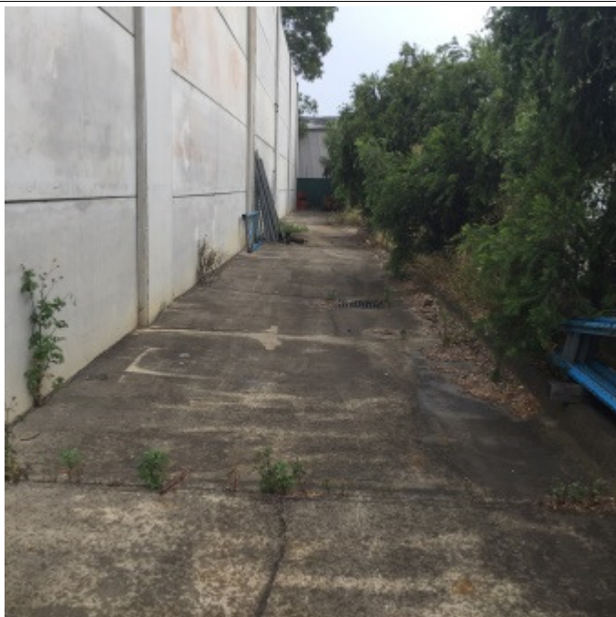
Photo 5.1.8 Concrete hardstand external to building
