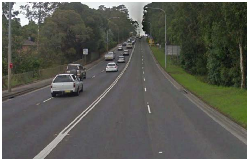
Figure 3-6 Princes Highway looking south (Source: Google)
