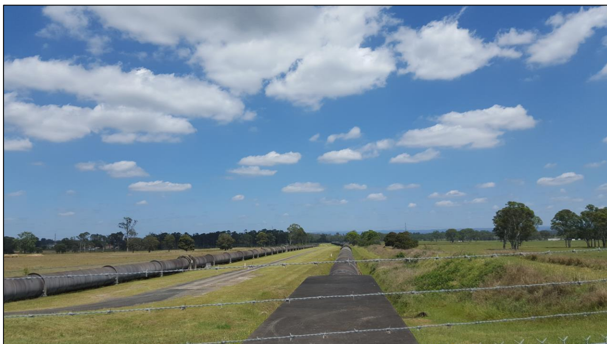
Photograph 4: View of managed easement to south of site
