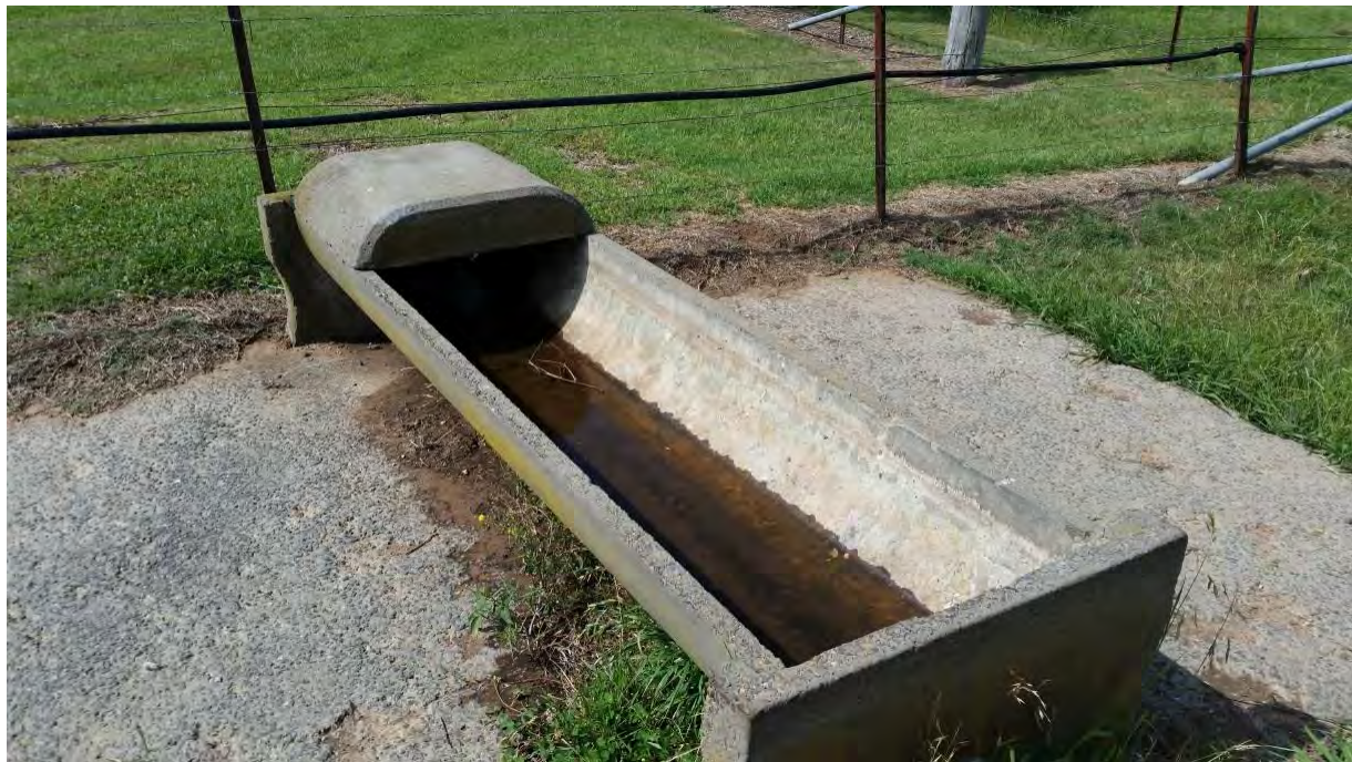
Site Photograph 6: Concrete trough located in the northwestern corner of the site.
