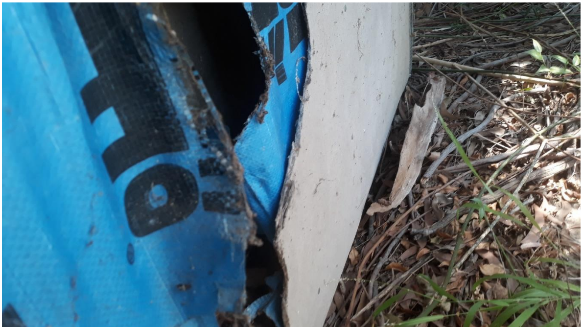
Photo 4: Exposed fibre board (potential ACM) 25 Mindarie St
