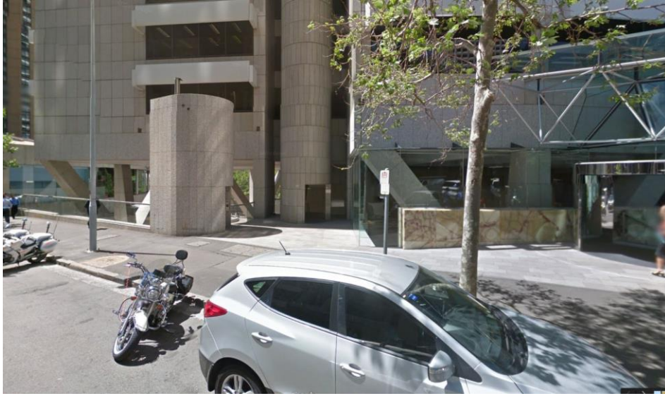
Figure 5 – Harrington Street entry of Grosvenor Place Source: Good Maps
