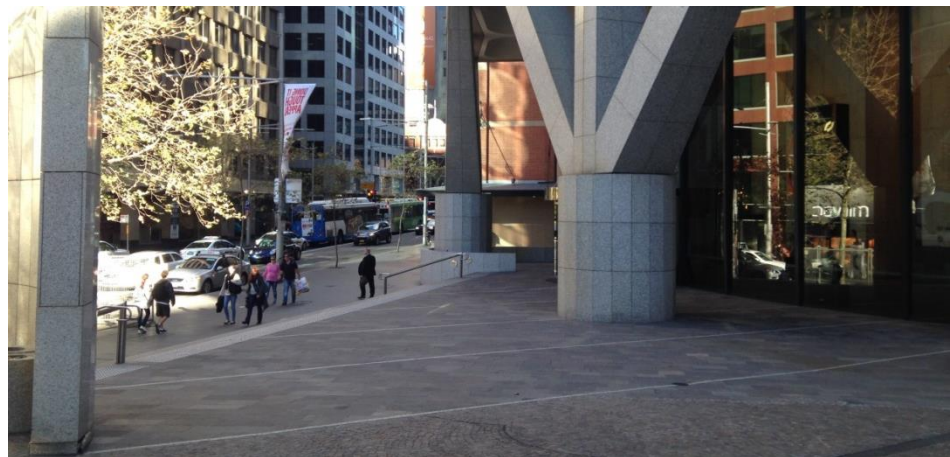
Figure 3 – George Street frontage of the forecourt Source: JBA
