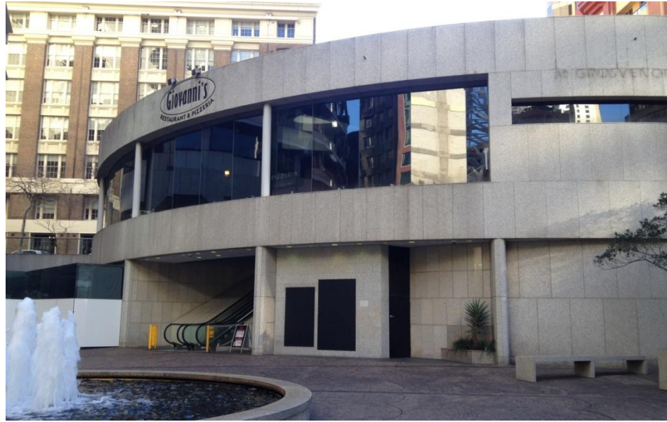
Figure 2 – North Court Building (prior to refurbishment) eastern facade Source: JBA
