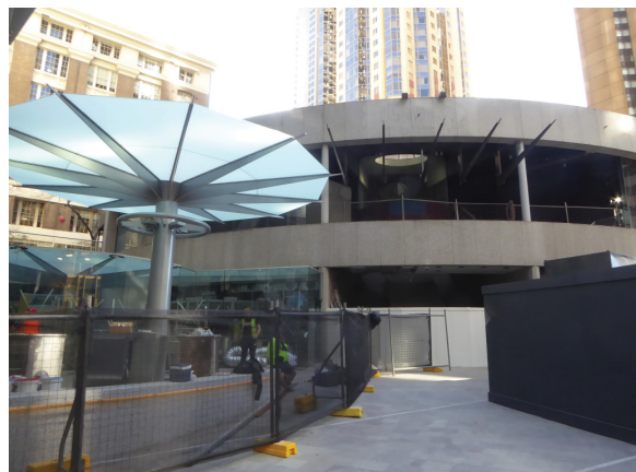
Figure 6: From the forecourt with the North Court building and an existing glazed canopy on the left
