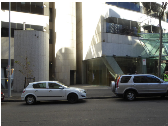
Figure 5: From Harrington Street with the lift drum on the left, the stairs beyond and glazed roof on the right
