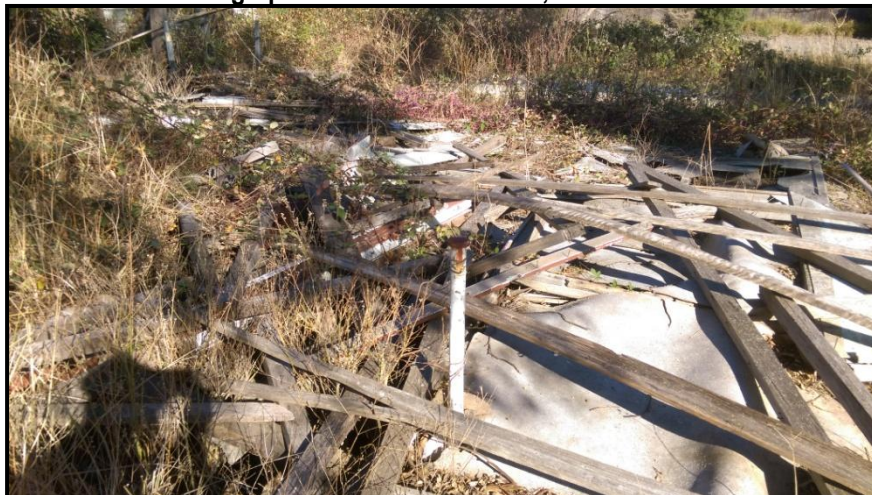
Photograph 5 – Demolition waste, west of house.
