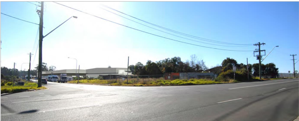
Picture 12 – Existing condition
