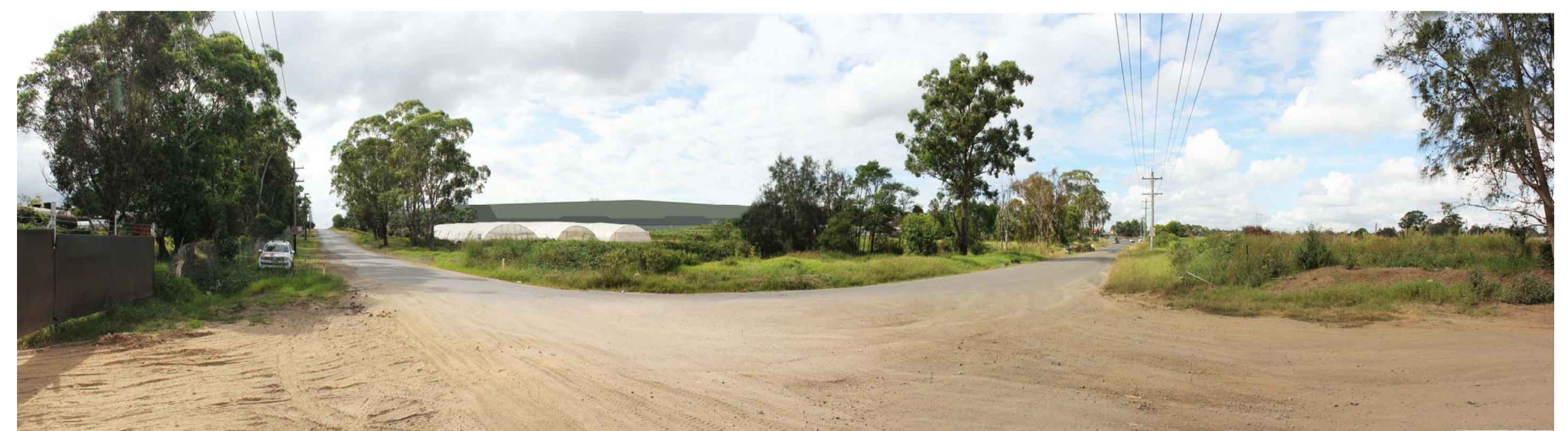
GROUND VIEW FROM NORTH WEST Cnr. YAURRUNGA STREET & KOOKABURRA ROAD NORTH
