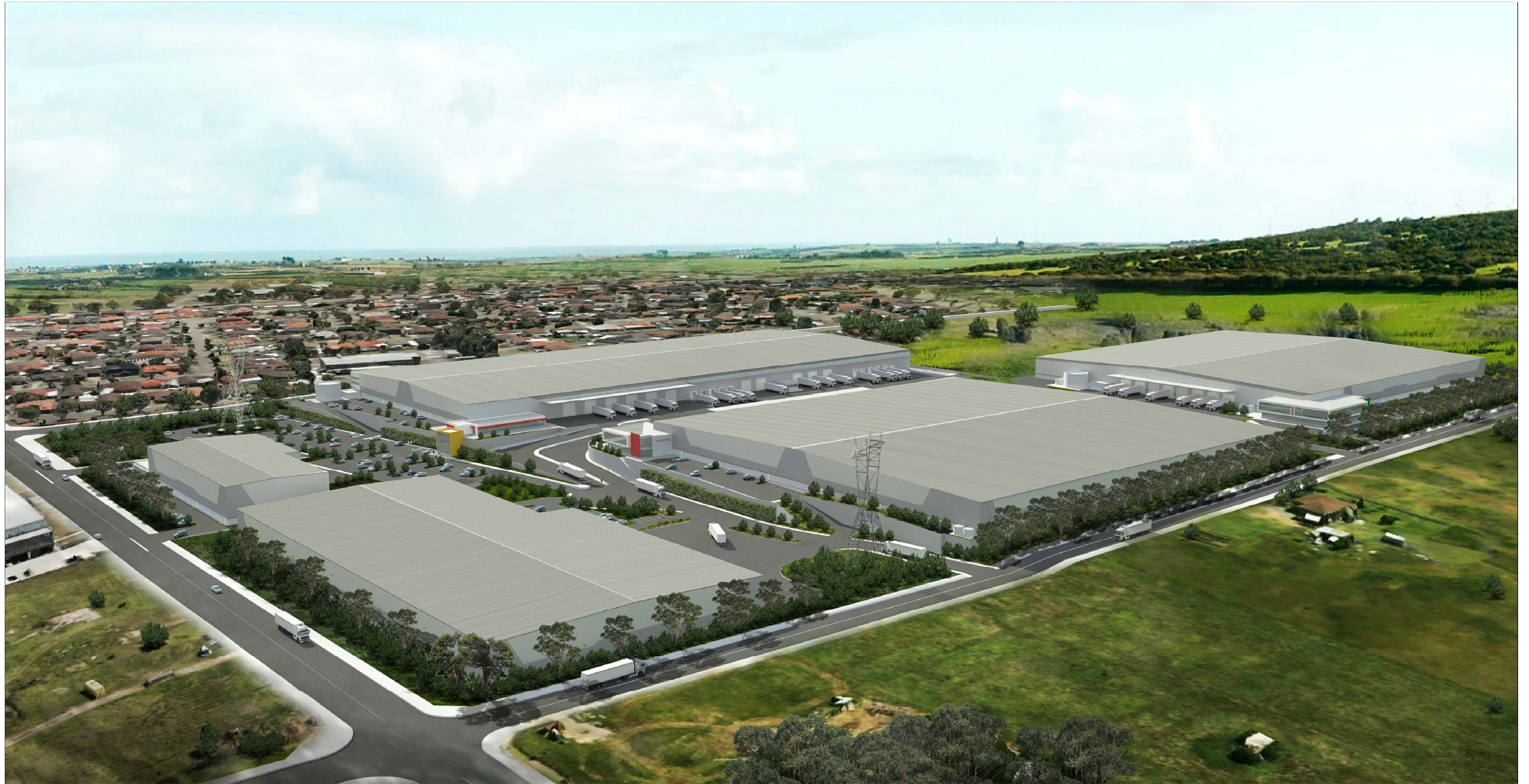
AERIAL VIEW FROM NORTH EAST
