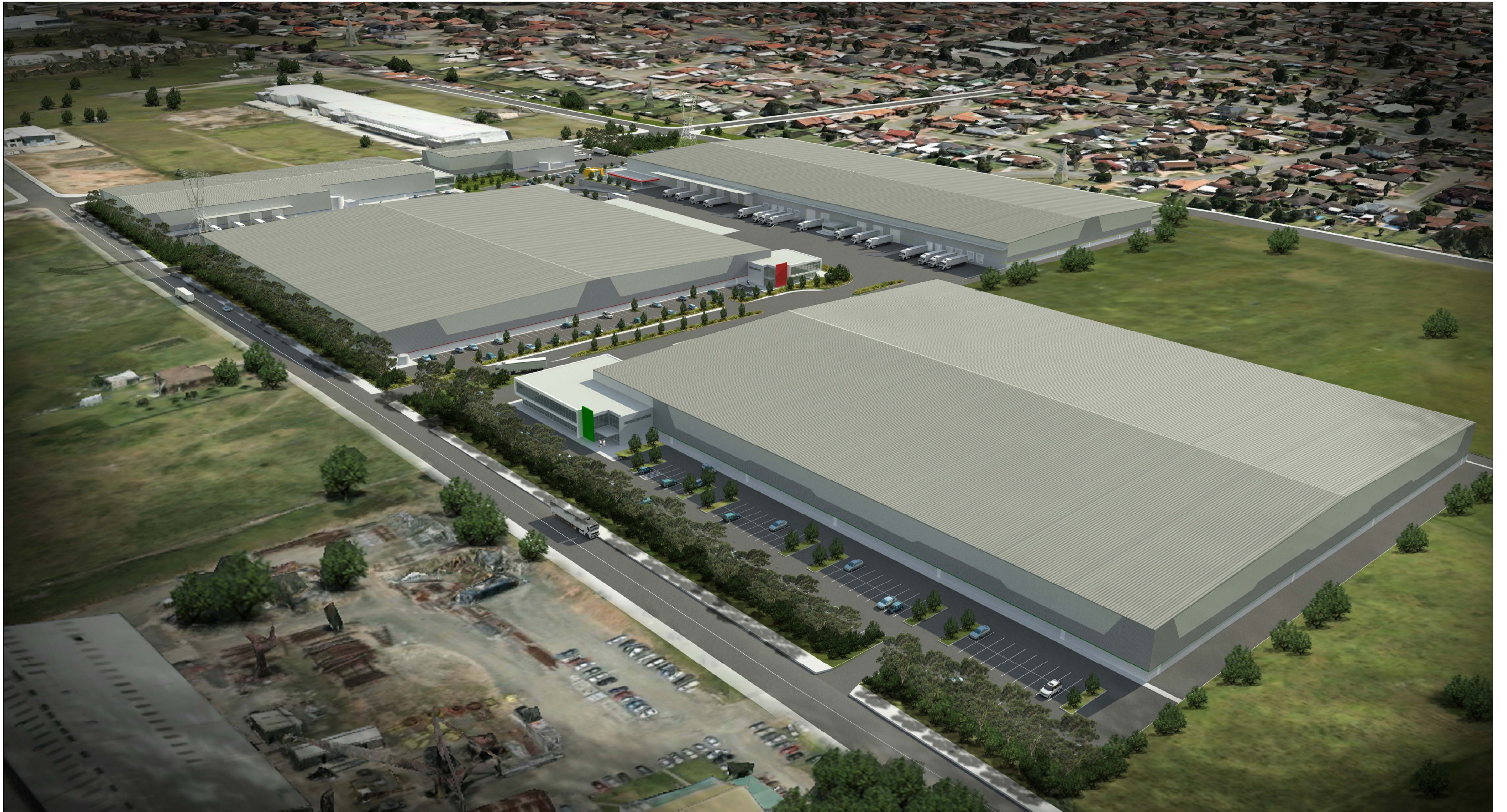
AERIAL VIEW FROM NORTH WEST
